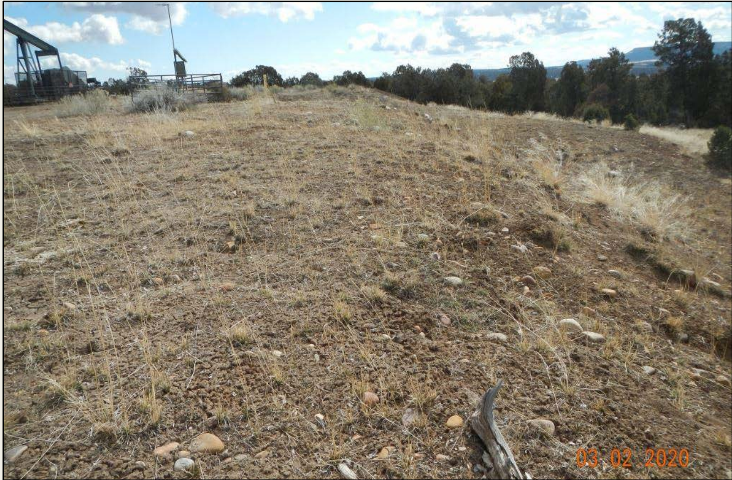
Photo 2. View of the southern fill slope facing eastward, revegetation is grazed but appears to be progressing with grasses such as sand dropseed and western wheatgrass.
