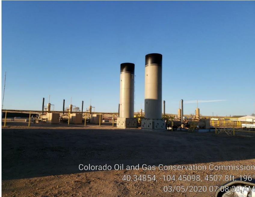
Photo #1 Separators & ECD's
