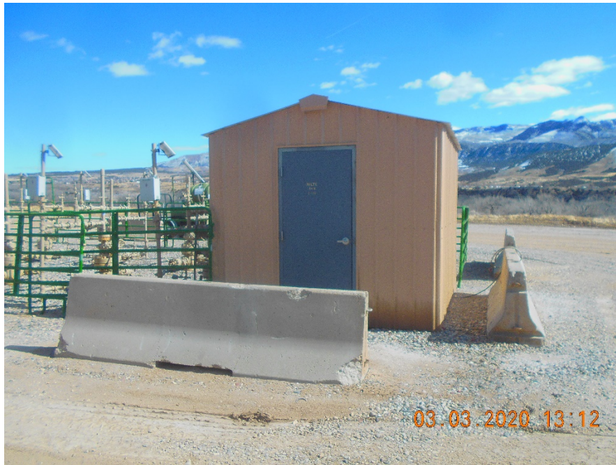
Injection wellhead housing with fence
