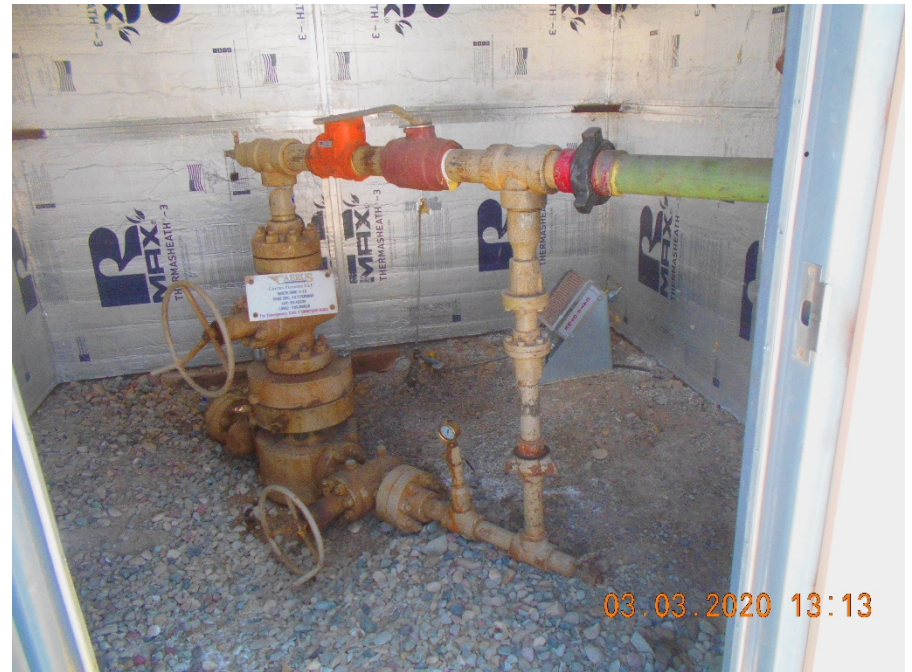
Wellhead flowline valves closed
