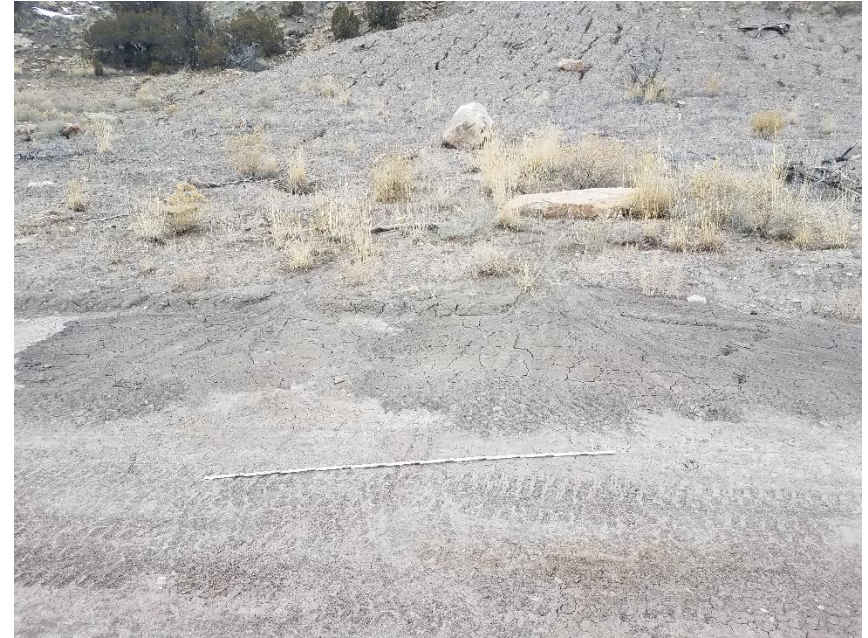
Photo 4: Photo taken from the access road, facing west. Photo shows sediment discharge from the Location onto the road. 6 foot measuring stick for reference.
