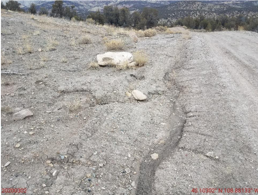
Photo 7: Photo taken from the access road, facing north. Photo shows stormwater runoff has caused degradation to the access road, and transported sediment off Location.
