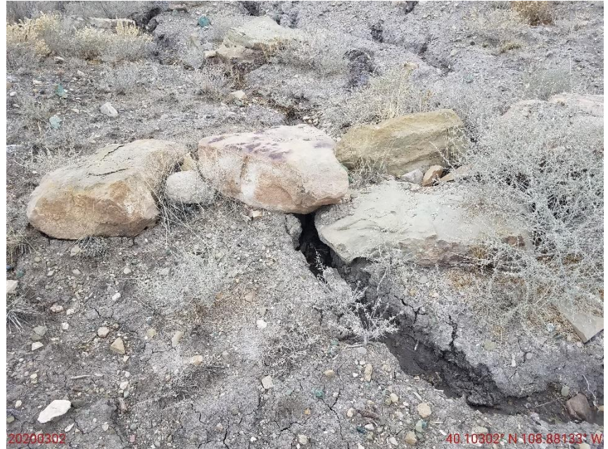
Photo 12: Photo taken from the Location, photo shows a rock-check documented in the previous inspection. Photo shows BMP has not been repaired or maintained in proper functioning condition, and installed in accordance with good engineering practices.
