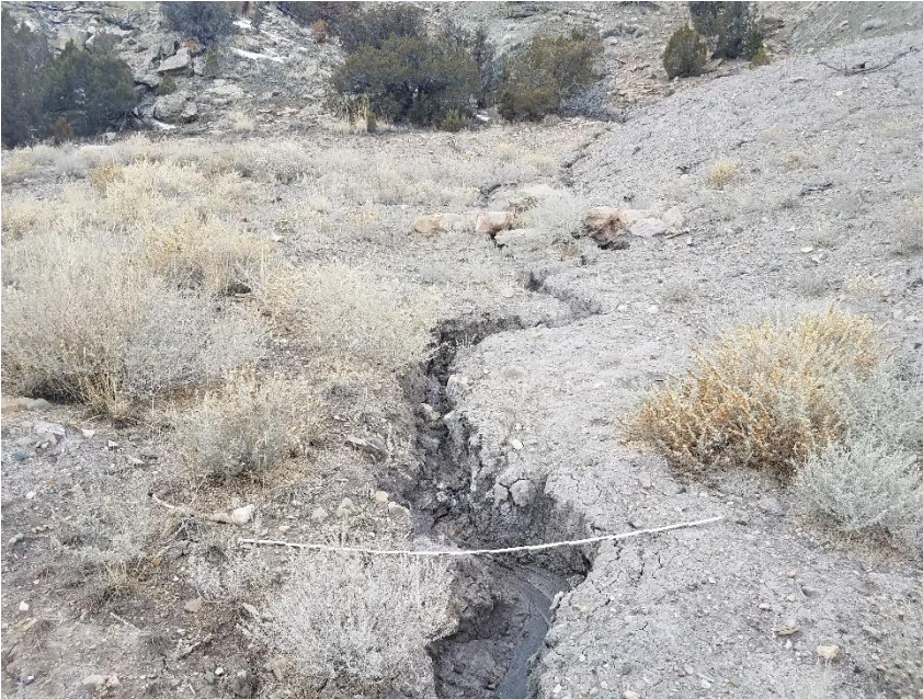
Photo 11: Photo taken from the Location, facing west. Photo shows gully erosion has not been repaired and stabilized, and stormwater BMPs have not been installed/maintained. 6 foot measuring stick for reference.
