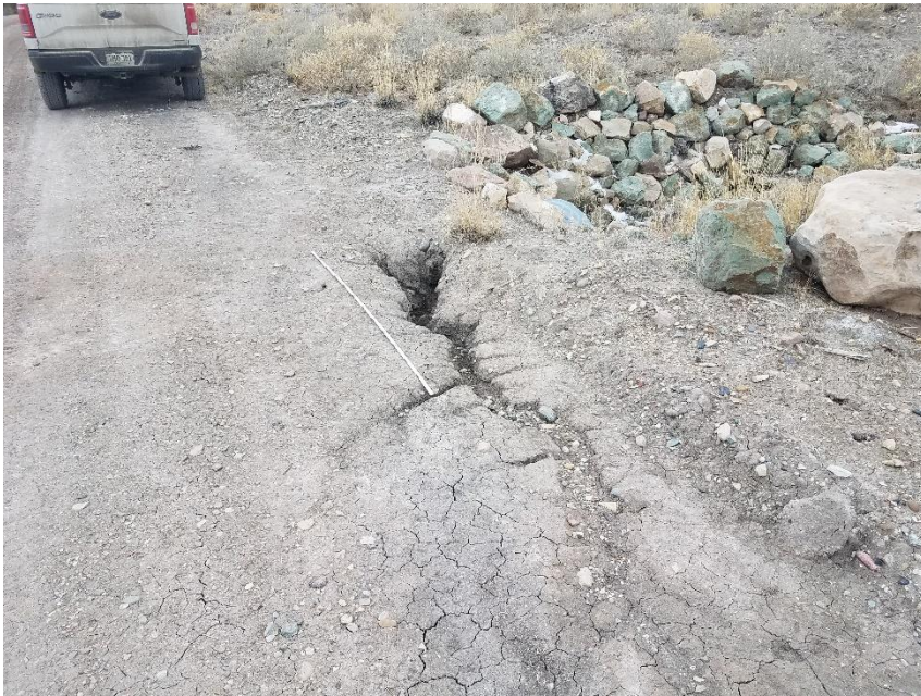
Photo 9: Photo taken from the access road, facing south. Photo shows stormwater erosion at access road has not been repaired/stabilized. Stormwater has continued to incise into the access road exposing the culvert. 6 foot measuring stick for reference.
