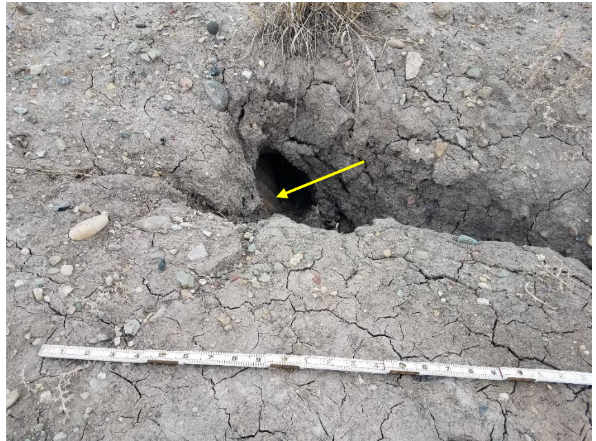
Photo 10: Continued from photo 9. Photo shows areas where Stormwater has continued to incise into the access road exposing the culvert (arrow).
