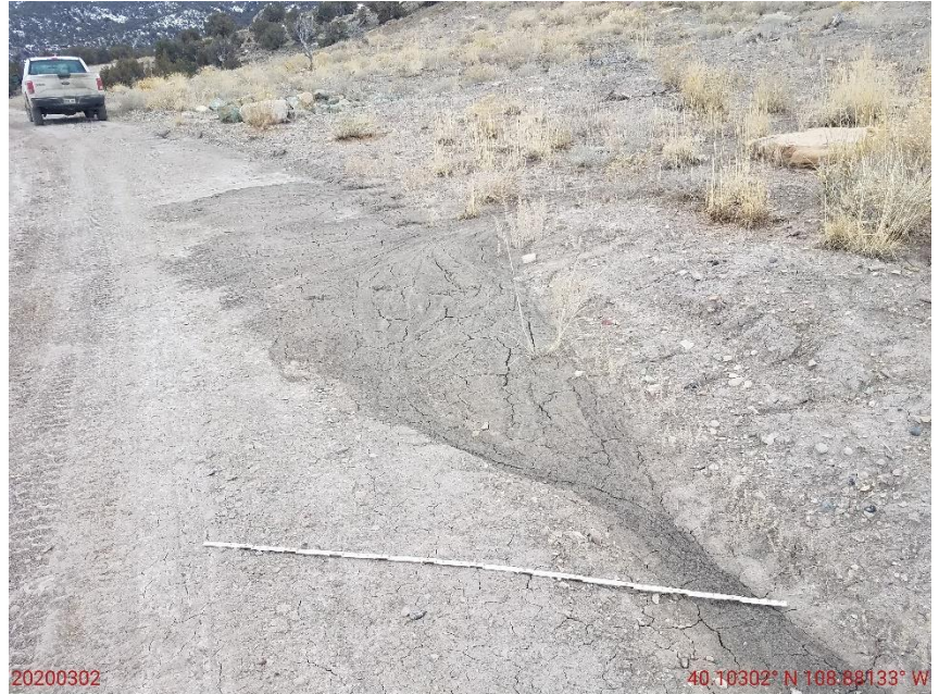
Photo 6: Photo taken from the access road, facing south. Photo shows sediment discharge from the Location onto the road. 6 foot measuring stick for reference.
