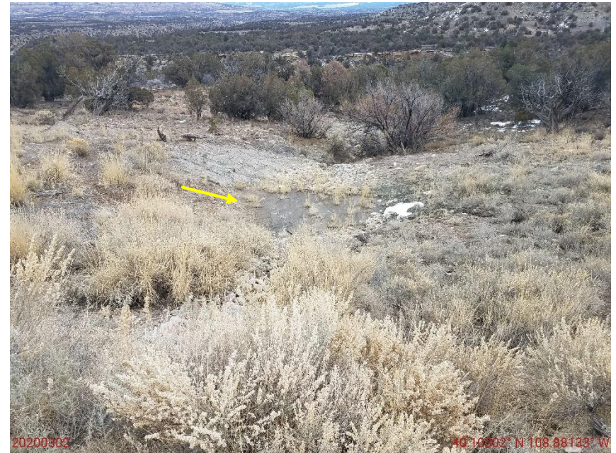
Photo 14: Photo taken from the east end of the location, facing east. Photo shows sediment trap has not been maintained and has filled with sediment due to sediment laden stormwater discharge.
