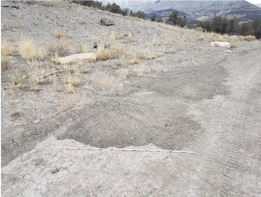
Photo 5: Photo taken from the access road, facing north. Photo shows sediment discharge from the Location onto the road. 6 foot measuring stick for reference.
