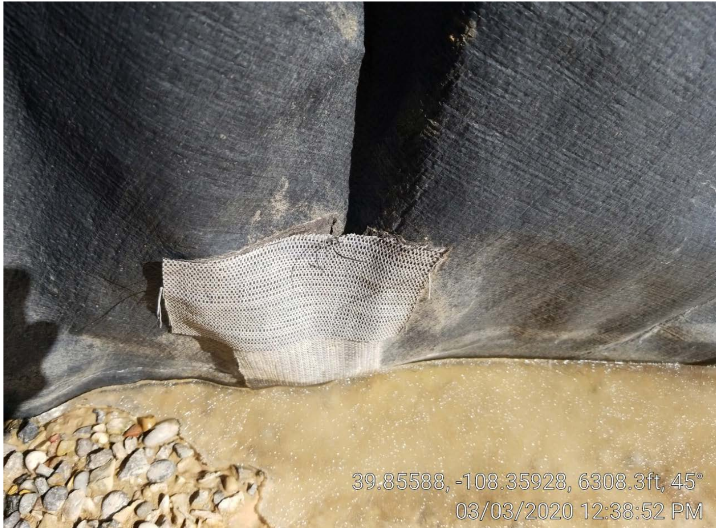
Photo 5. Loose liner patch.
