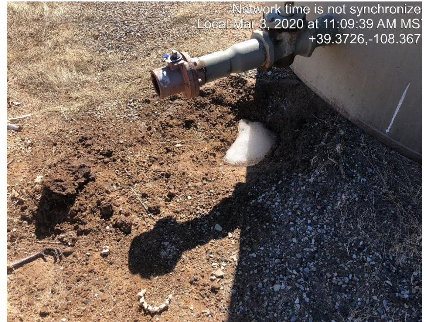
Photo #0683 Stained soils under load out valve on tank.
