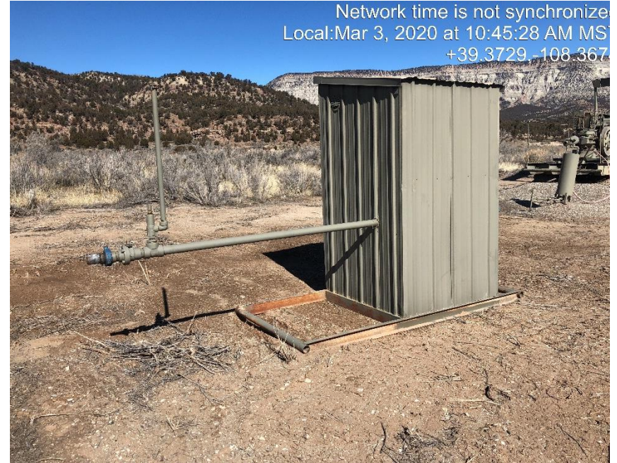
Photo #0679 Unused meter run.
