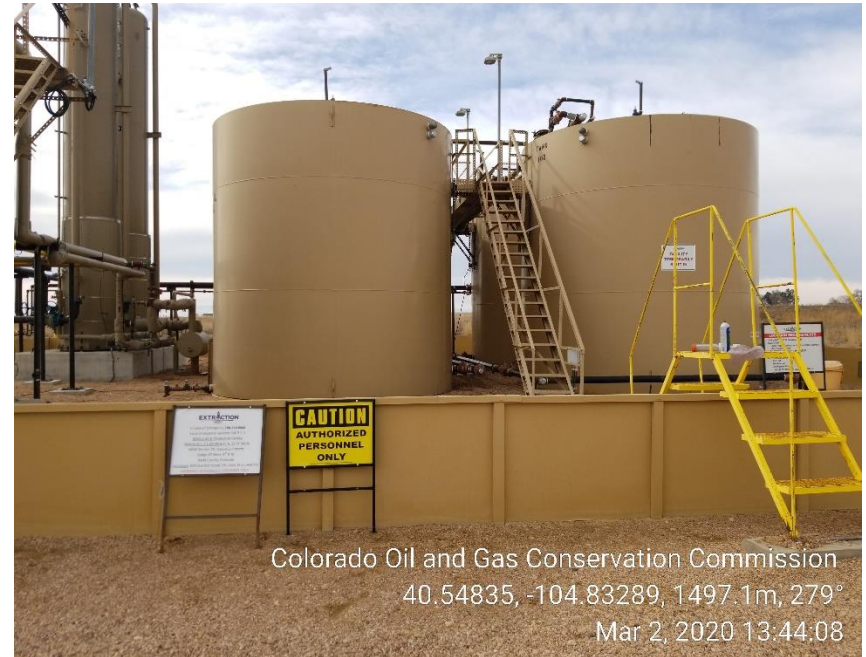
Photo 18: Tank Battery
