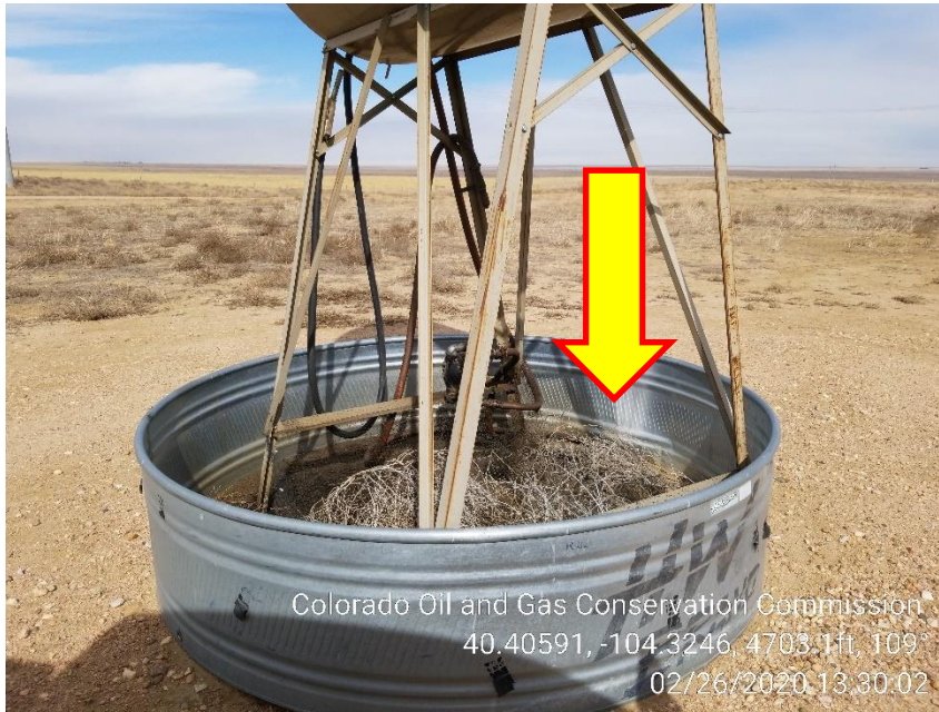
Photo 3 – Debris inside containment, Wildlife netting in disrepair.
