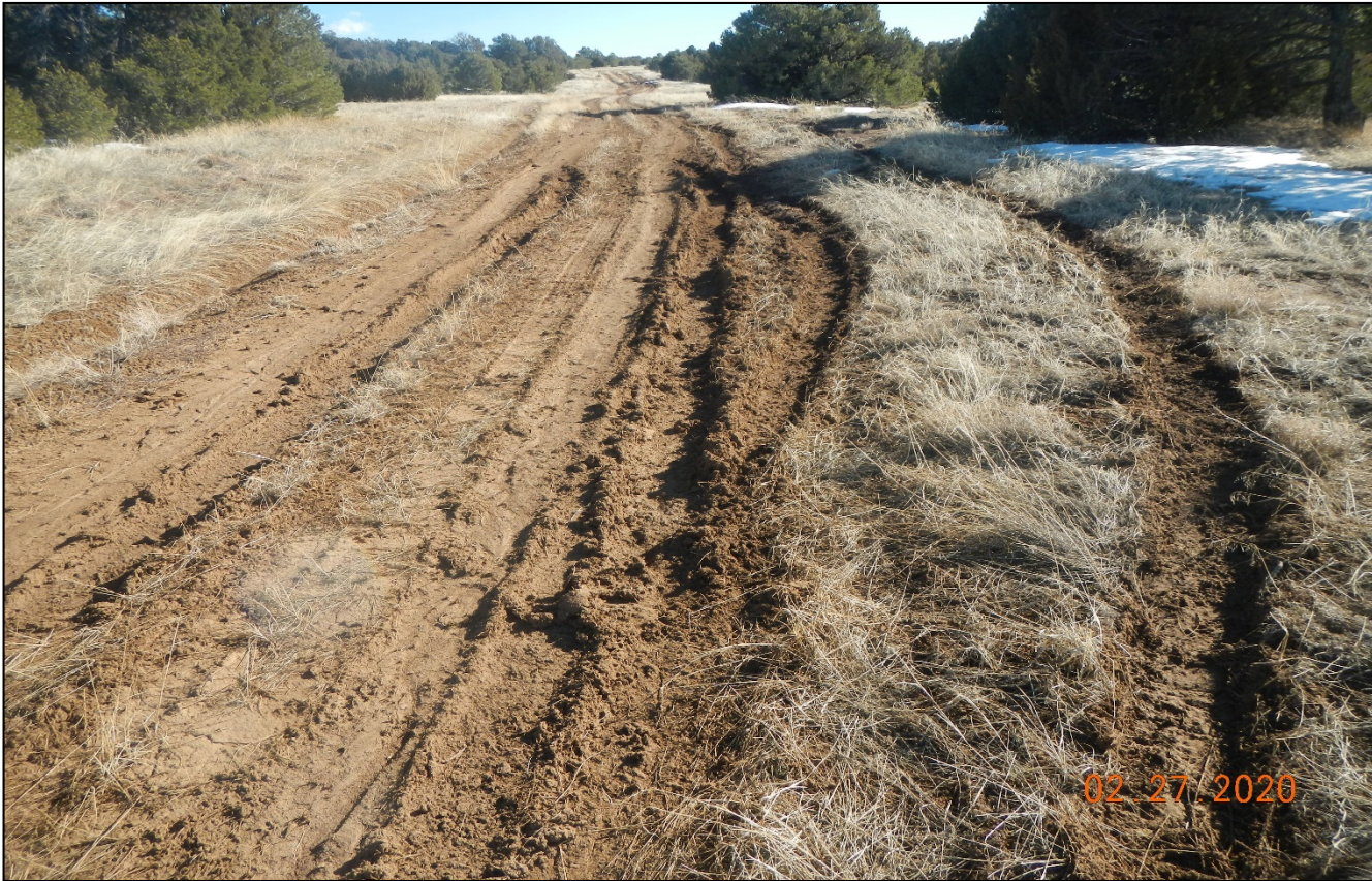
Photo 4. Vehicle use of the road during wet conditions is causing ruts and damage along the road.
