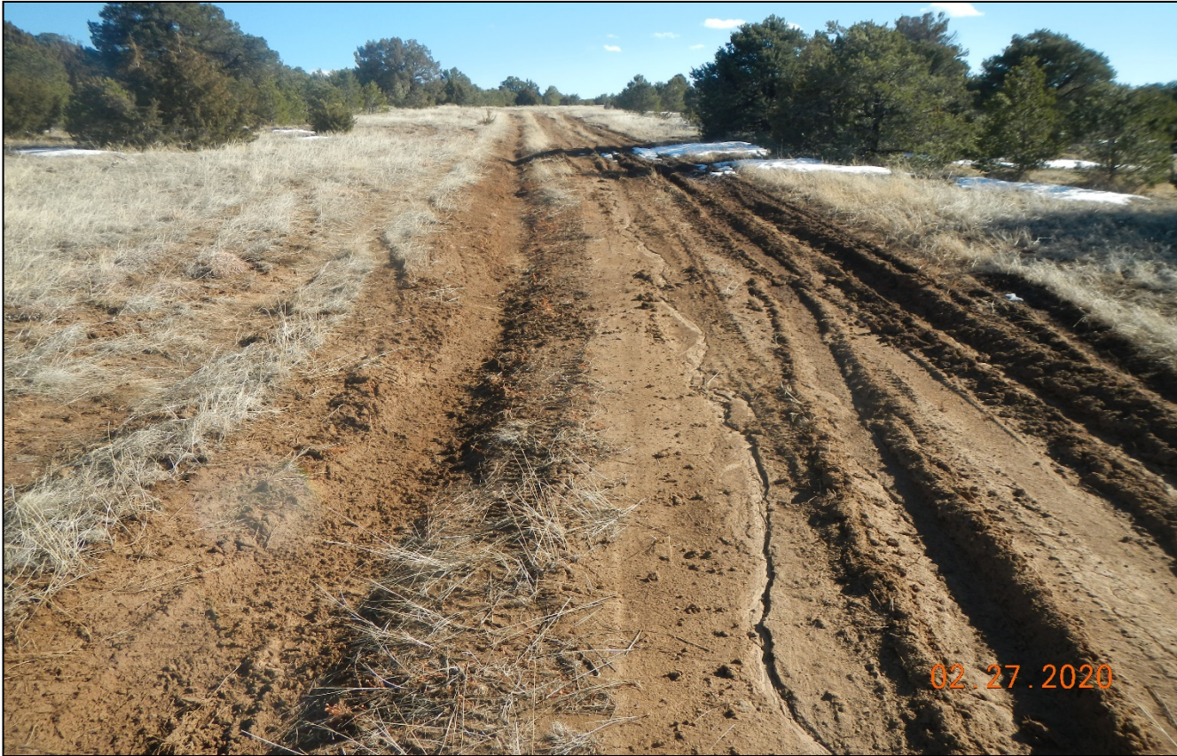
Photo 5. Vehicle use of the road during wet conditions is causing ruts and damage along the road.
