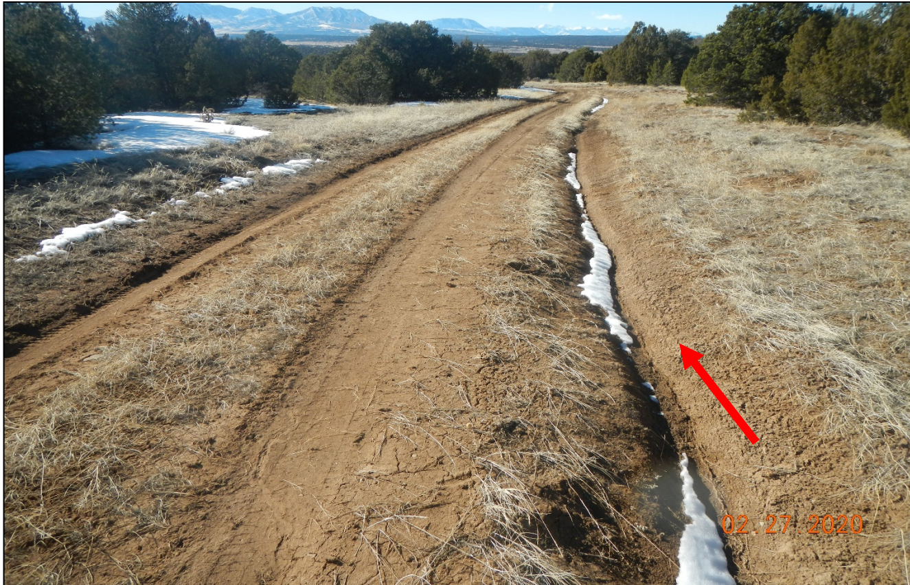
Photo 3. The side of the road has no BMP's installed to prevent erosion. The long downward grade of the road will accelerate stormwater and may deepen the side shown by red arrow.
