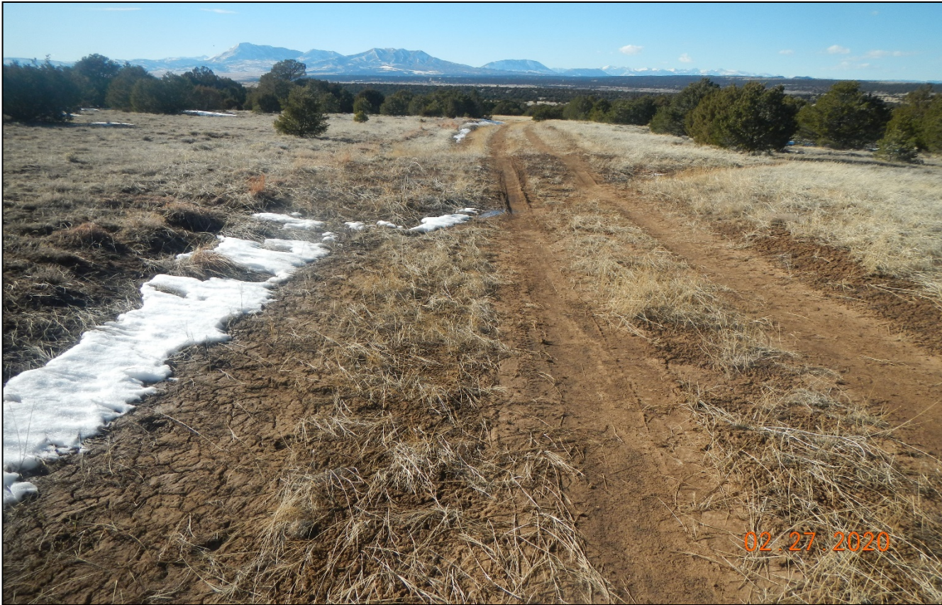
Photo 8. Facing northwest along the access road. Vegetation appears to be establishing along the side of the road. Vehicle rutting is not occurring in this area.
