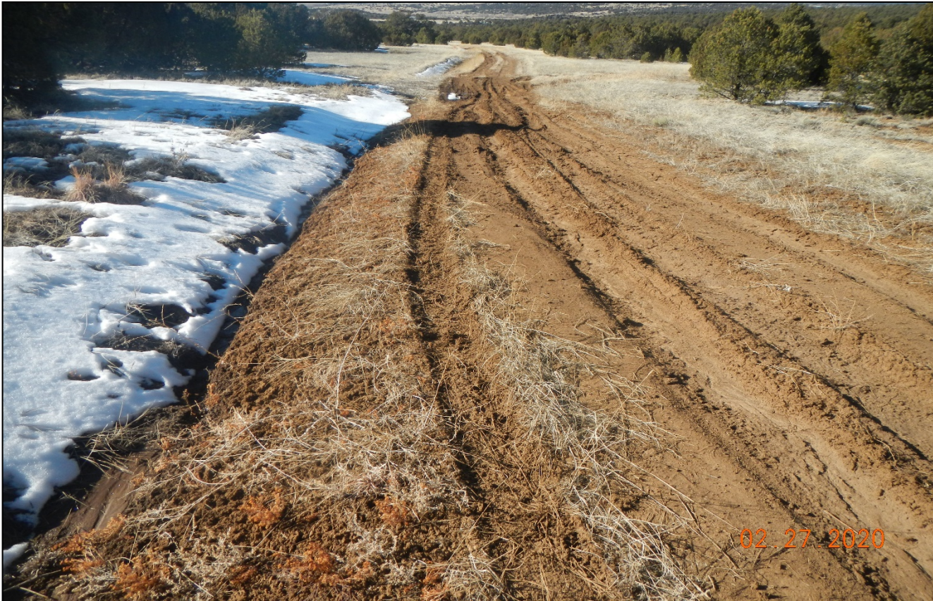
Photo 6. Facing northwest along the access road. The long downward grade of the road could accelerate stormwater along the side of the road and also along the vehicle ruts.
