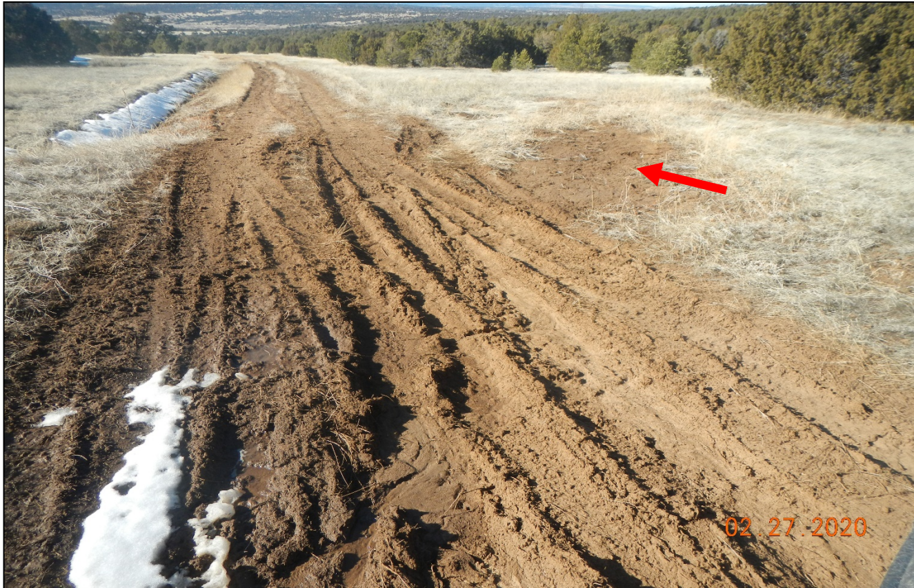
Photo 7. Facing northwest along the road at the water bar. It appears sediment is accumulating at outlet (red arrow). This may cause stormwater to flow over the water bar and down the road. A sediment trap or other BMP may be needed at the end of the water bar outlet.
