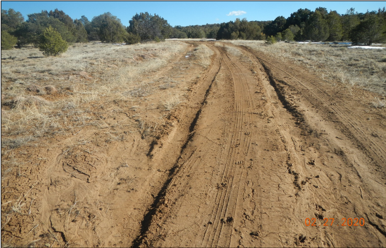
Photo 2. There is vehicle rutting along the road. The ruts will cause stormwater to flow down along the ruts and could cause erosion.
