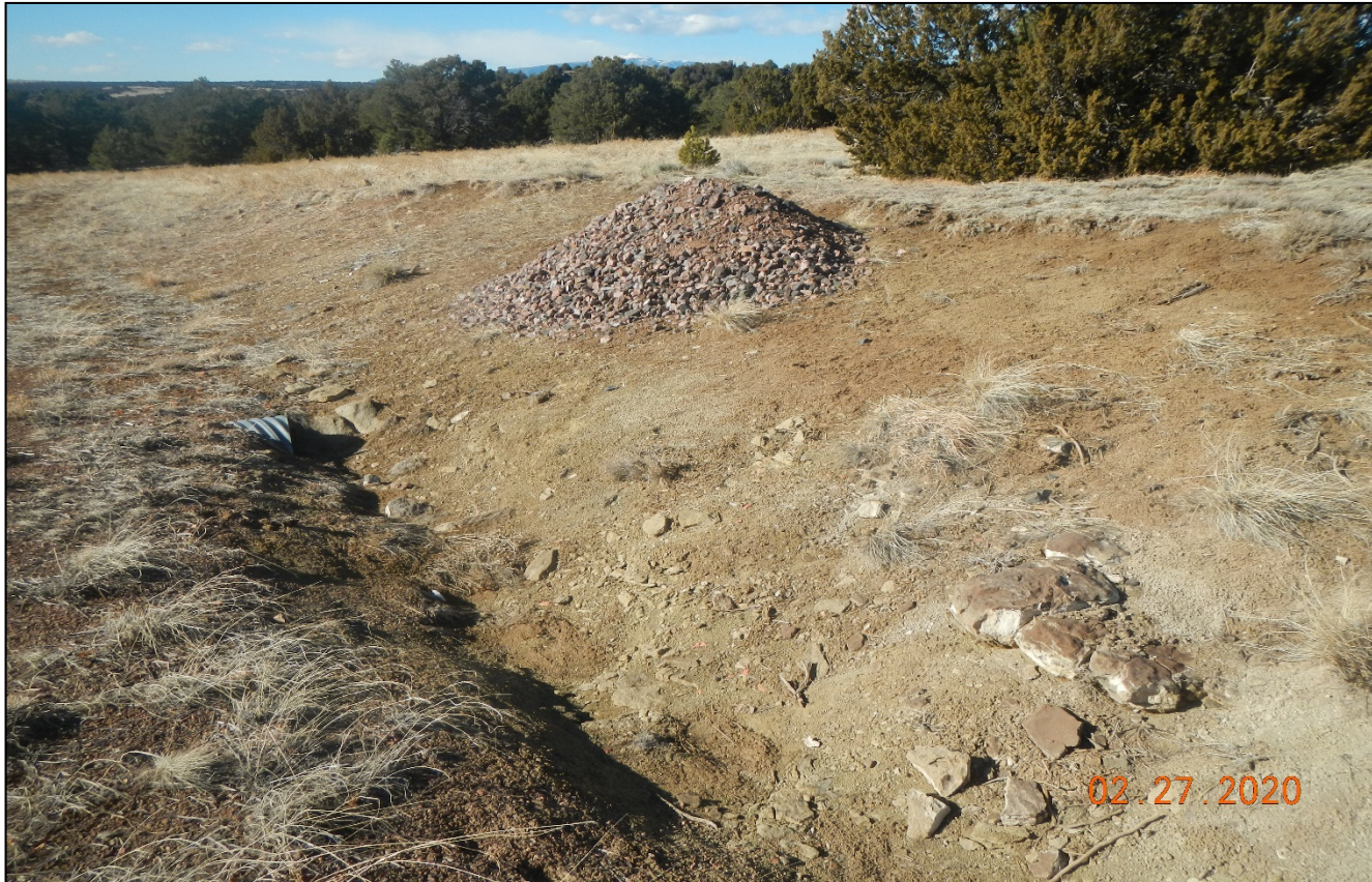
Photo 2. This cut slope area near the culvert does not have adequate vegetation establishment. There is a pile of rock left at the slope.
