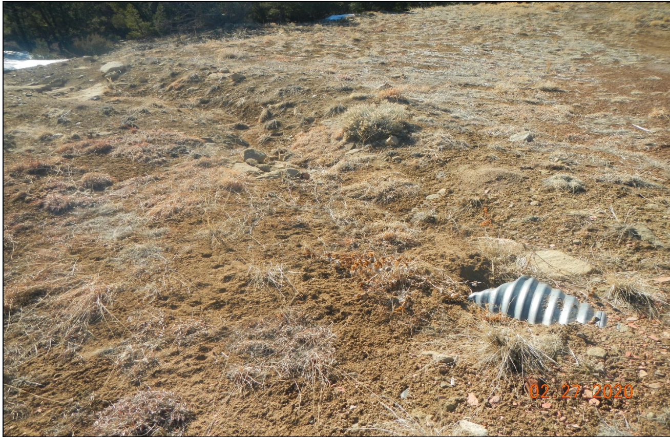
Photo 3. The outlet culvert has filled in with sediment. A sediment trap may be need at culvert outlet.
