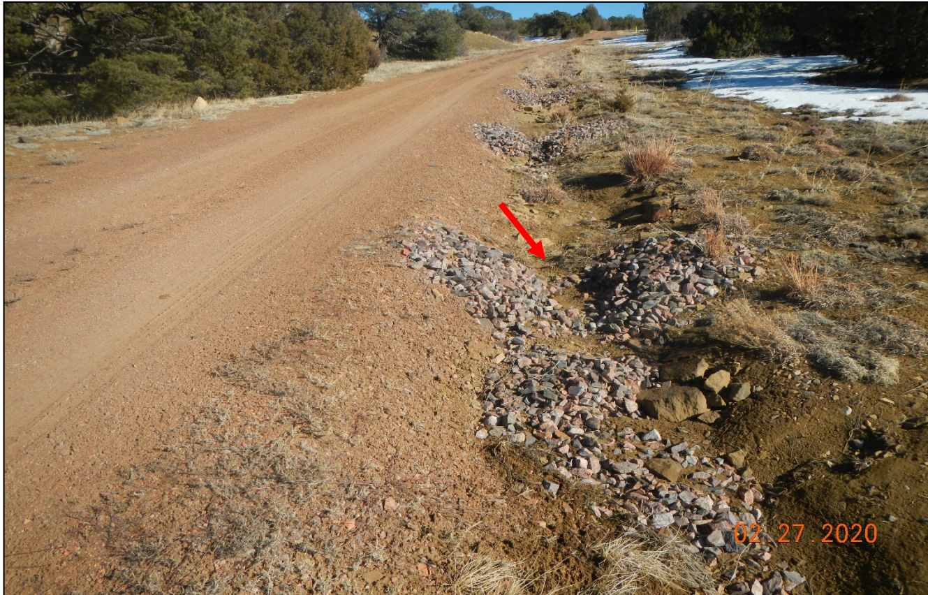
Photo 1. Facing southeast along the access road. Rock check dams were installed along the side of the road but have since failed. The rock has been displaced as shown by arrow.
