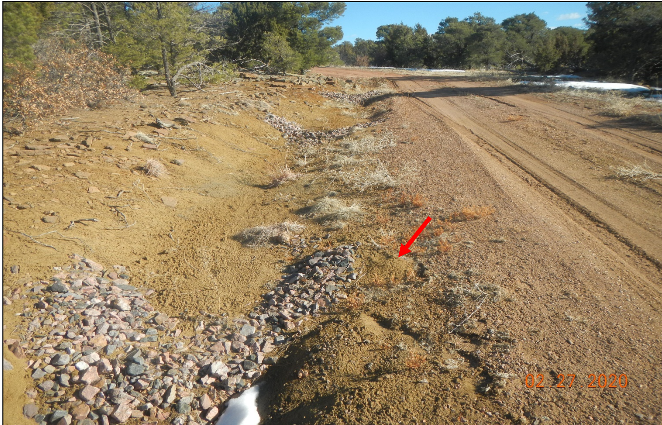
Photo 3. The check dams have filled in with sediment and are starting to erode around the check dam shown by arrow. The side of road should be seeded and stabilized.
