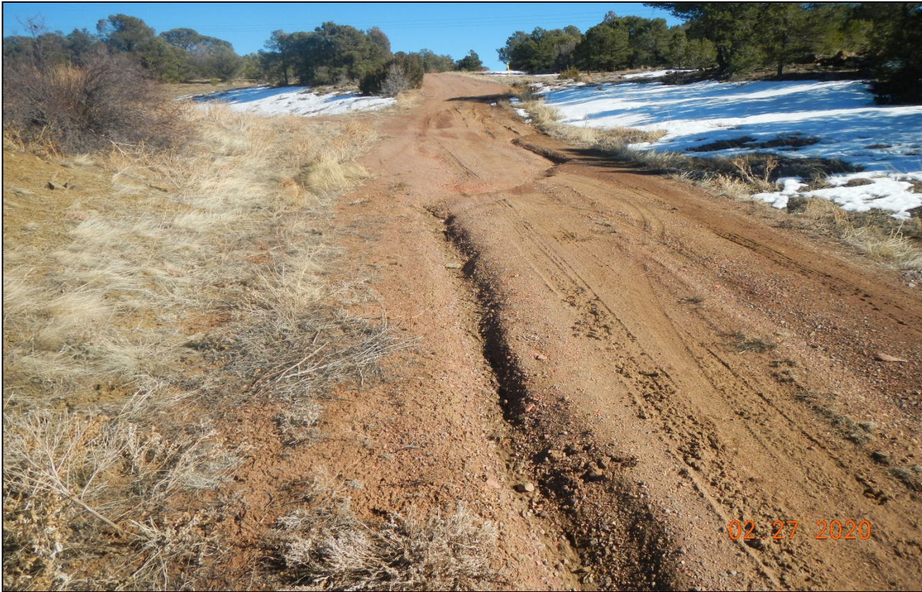
Photo 2. Stormwater is flowing down the road causing erosion near the State 7W location.
