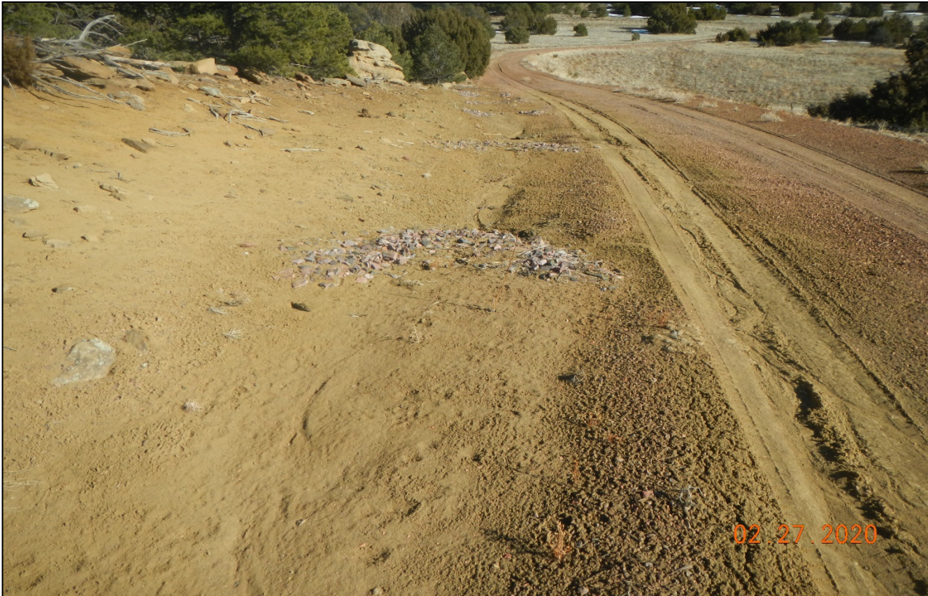
Photo 8. Facing southeast at the south side of the location. The access road continues toward the State 10WB. This check damn has filled in with sediment. The side of road should be seeded and stabilized.
