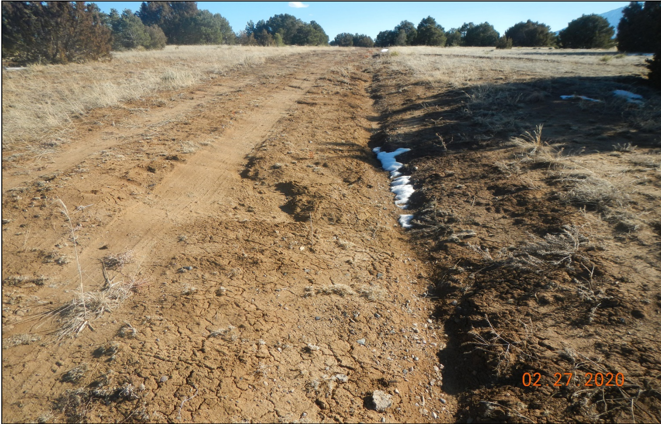
Photo 2. There is an erosion channel along the former road. This needs to be repaired and reclaimed.
