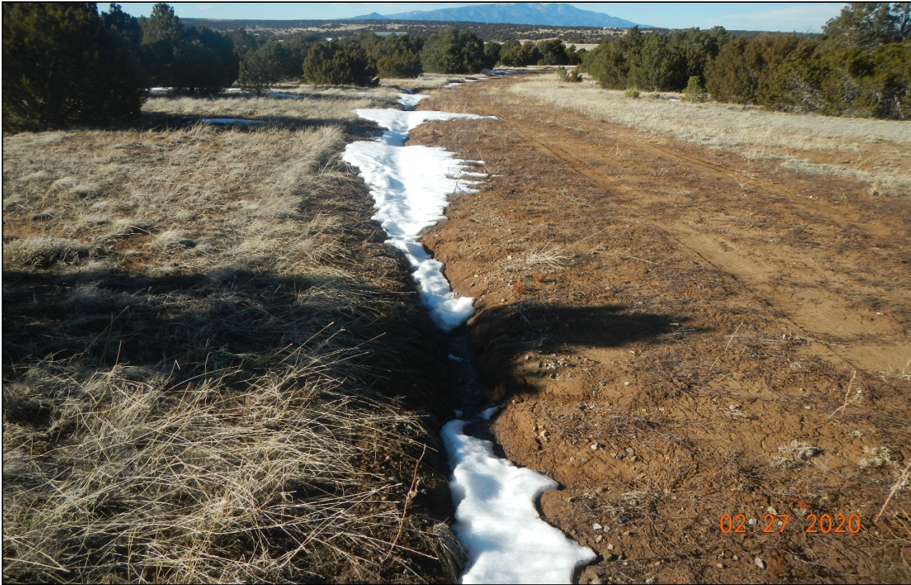
Photo 3. Facing back north toward the road. An erosion channel has formed along and vegetation has not established along the road.
