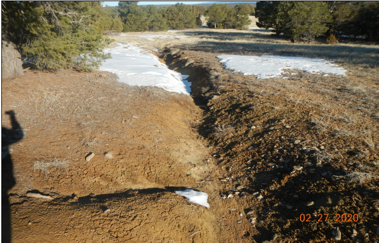
Photo 3. This erosion channel along the access road needs to be repaired and stabilized with vegetation. This channel needs to be filled in and reclaimed.
