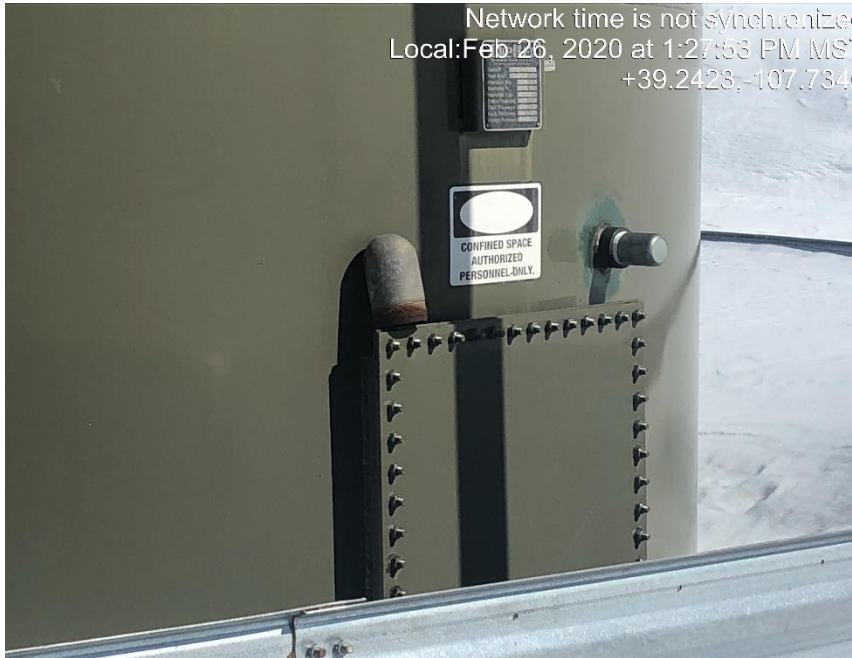
Photo #0651 Multiple unused bull plugs on top of tank man way covers.
