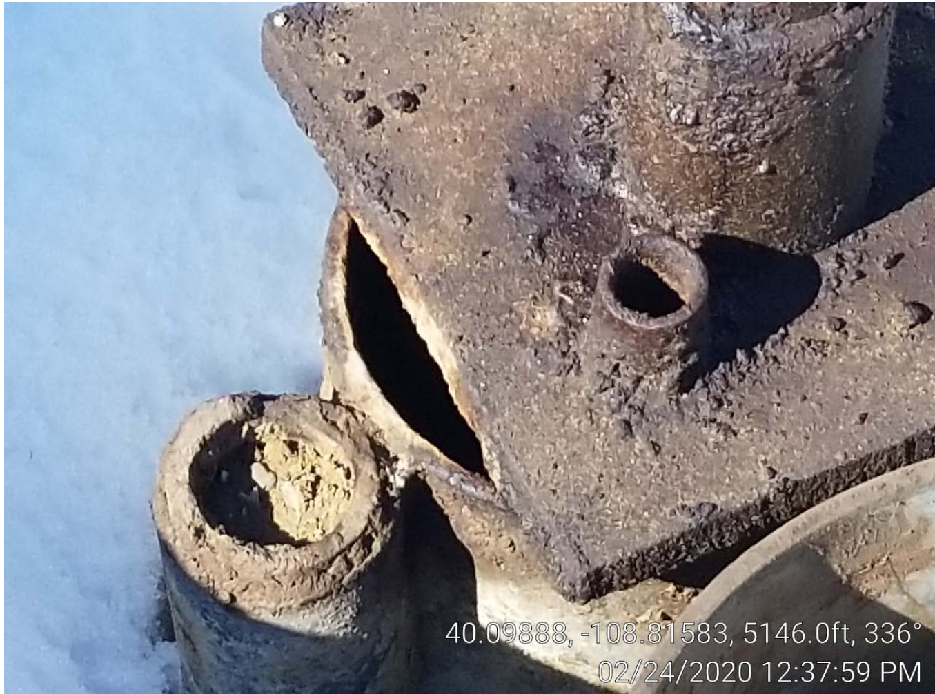
Photo 7. Casing open to atmosphere well Stagner 6.
