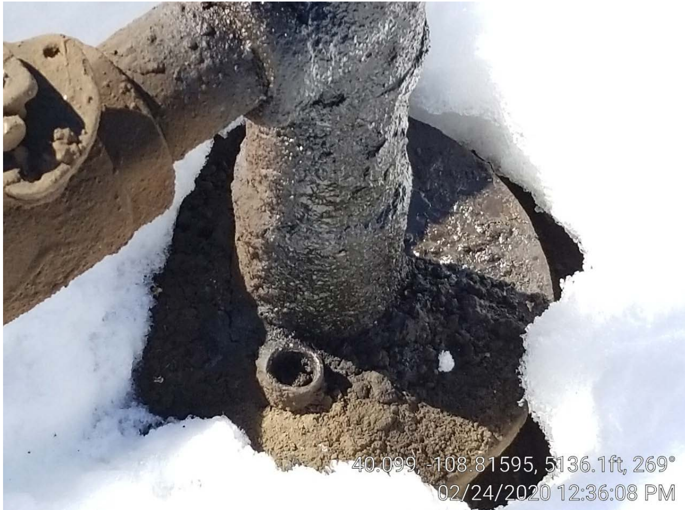
Photo 3. Hole on top of casing of well Stagner 2.
