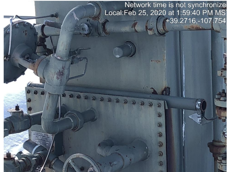
Photo #0641 Unused 2" pipe on separator.
