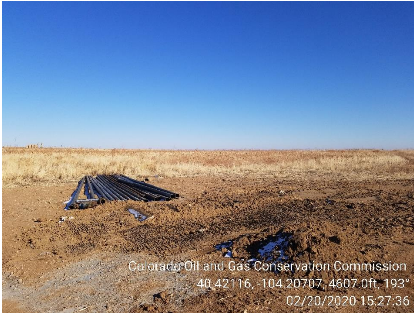
Photo 1 – Well recently Plugged and Abandoned. Unused Casing and Wellhead parts still on location
