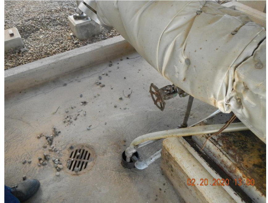
Secondary containment and sump drain.
