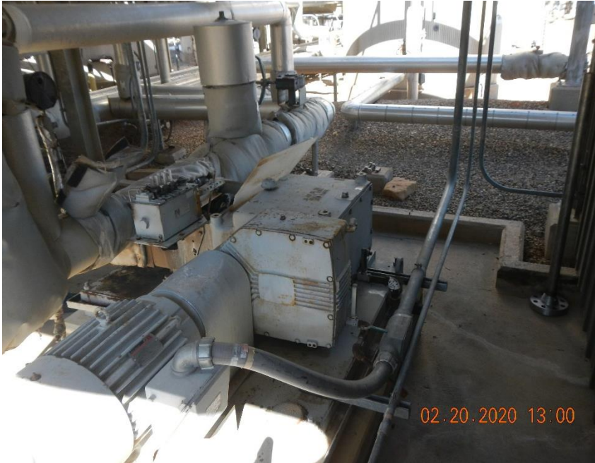
Packing failed on produced water pump.
