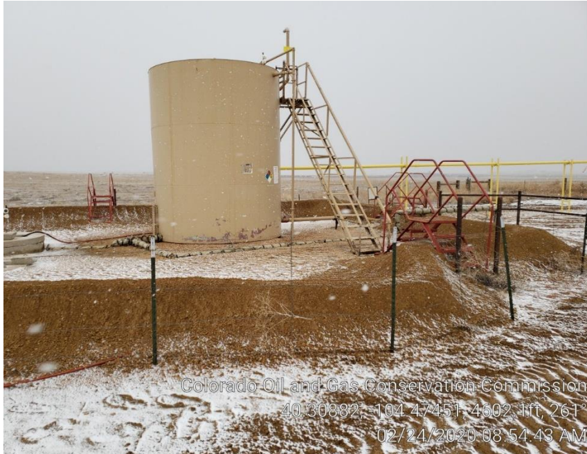
Photo #3 Tank Battery & Adequate Berm
