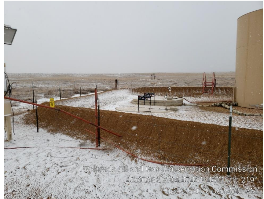
Photo #2 Adequate Berm
