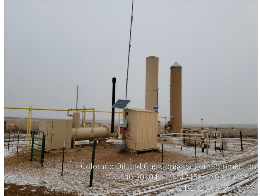
Photo #4 Separator, ECD's & Meter Run
