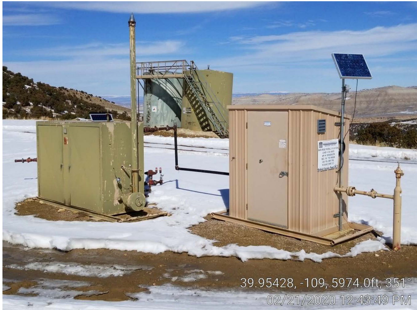
Photo 3. Separator, tanks, meter building.
