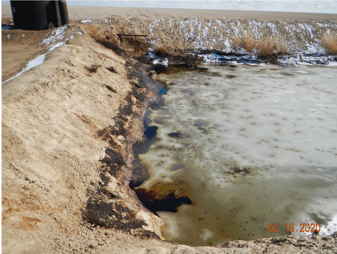
Photo # 2 – Oily soil on pit bank, oil on surface of pit
