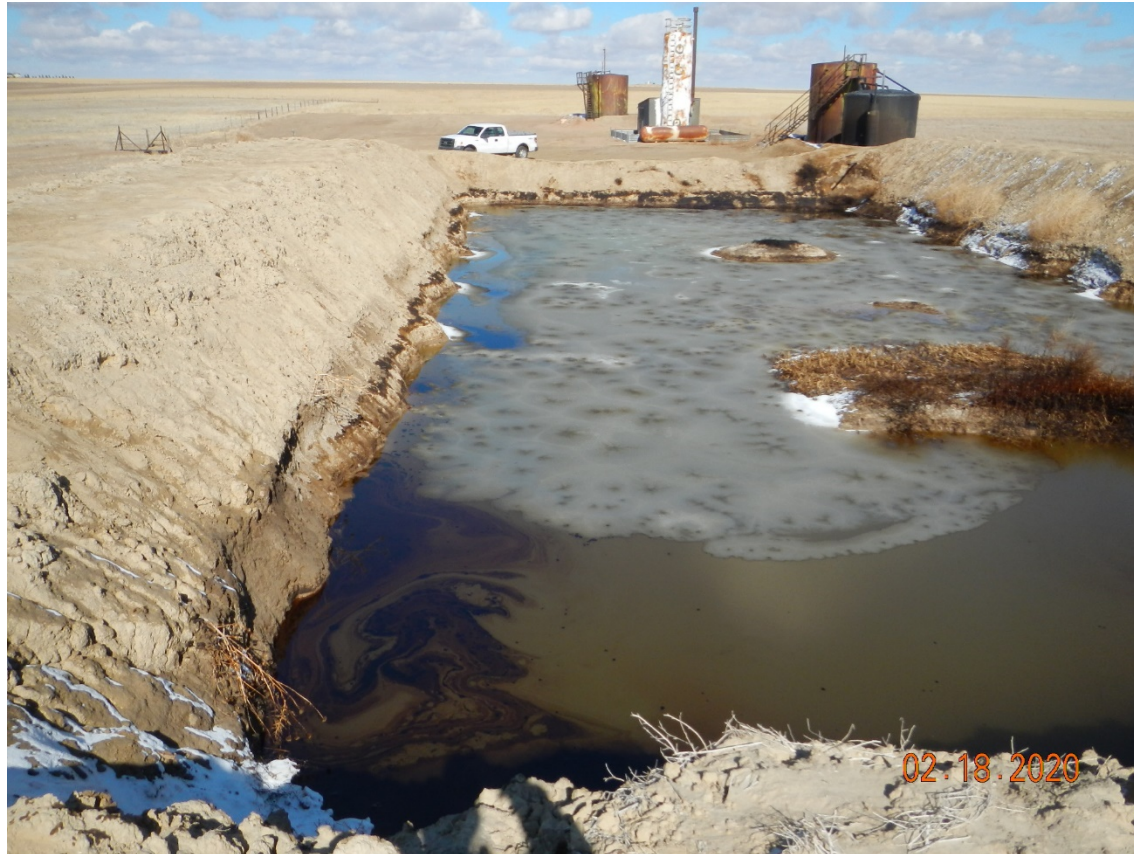
Photo # 5 – View north at pit with oil on the surface, oil on pit berms in northeast corner
