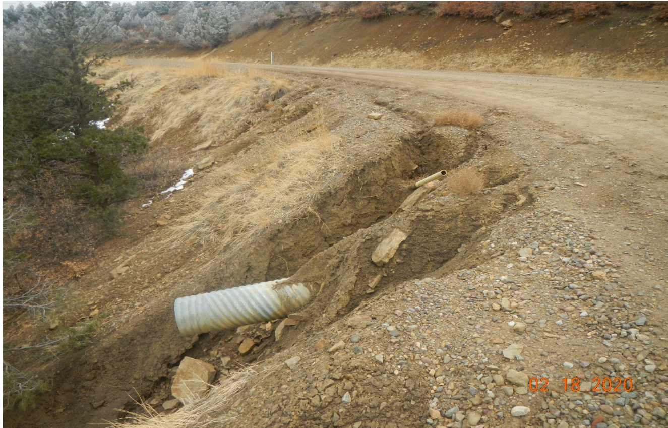
Photo 5. Stormwater runoff from the road is causing erosion near this culvert at Lat/Long:37.05297,-104.82619. There is no outlet protection installed at the culvert outlet.
