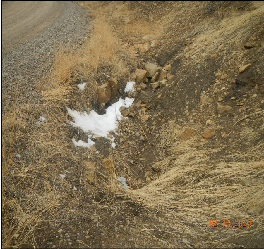
Photo 3. The above photos of the culvert inlet and outlet were taken at Lat/Long:37.05354,-104.82491. The inlet culvert has filled in with sediment and the outlet culvert is causing erosion.
