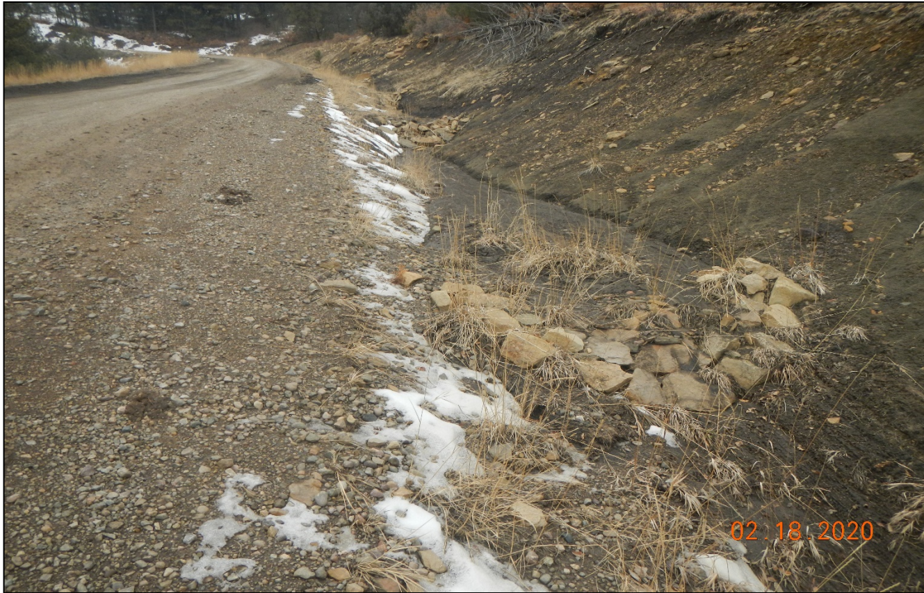
Photo 1. Erosion is occurring on the side of the road and rock check damns have filled up with sediment at Lat/Long:37.0586,-104.81750.
