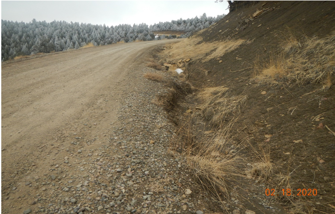
Photo 4. Facing southwest along the main lease road. Erosion is occurring along the side of the road.
