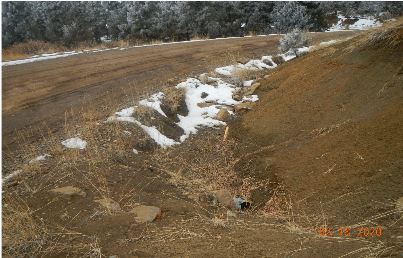
Photo 6. This culvert along the main road has filled in with sediment.
