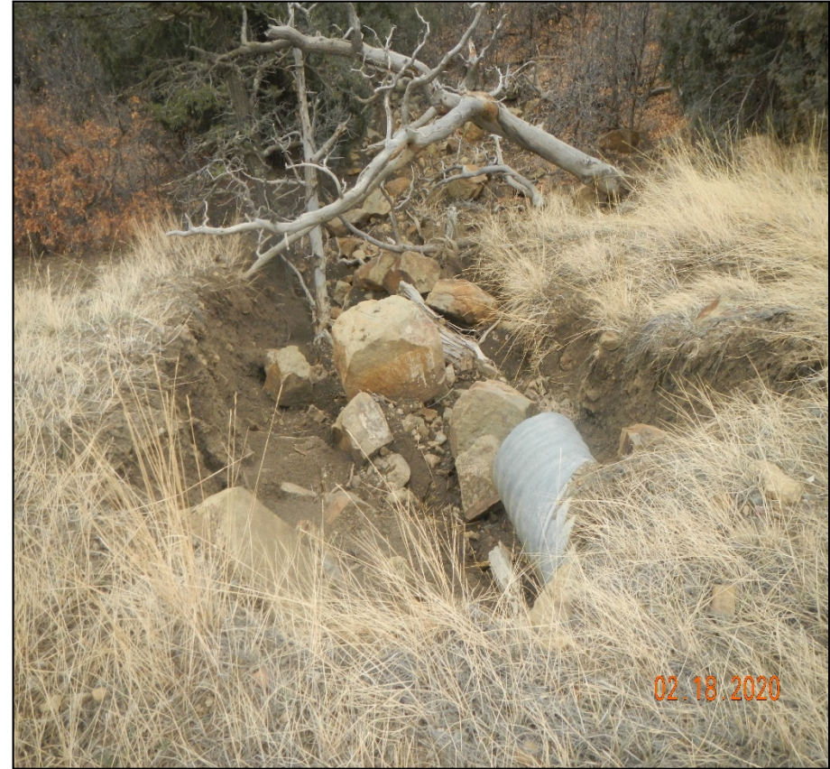
Photo 3. The above photos of the culvert inlet and outlet were taken at Lat/Long:37.05354,-104.82491. The inlet culvert has filled in with sediment and the outlet culvert is causing erosion.
