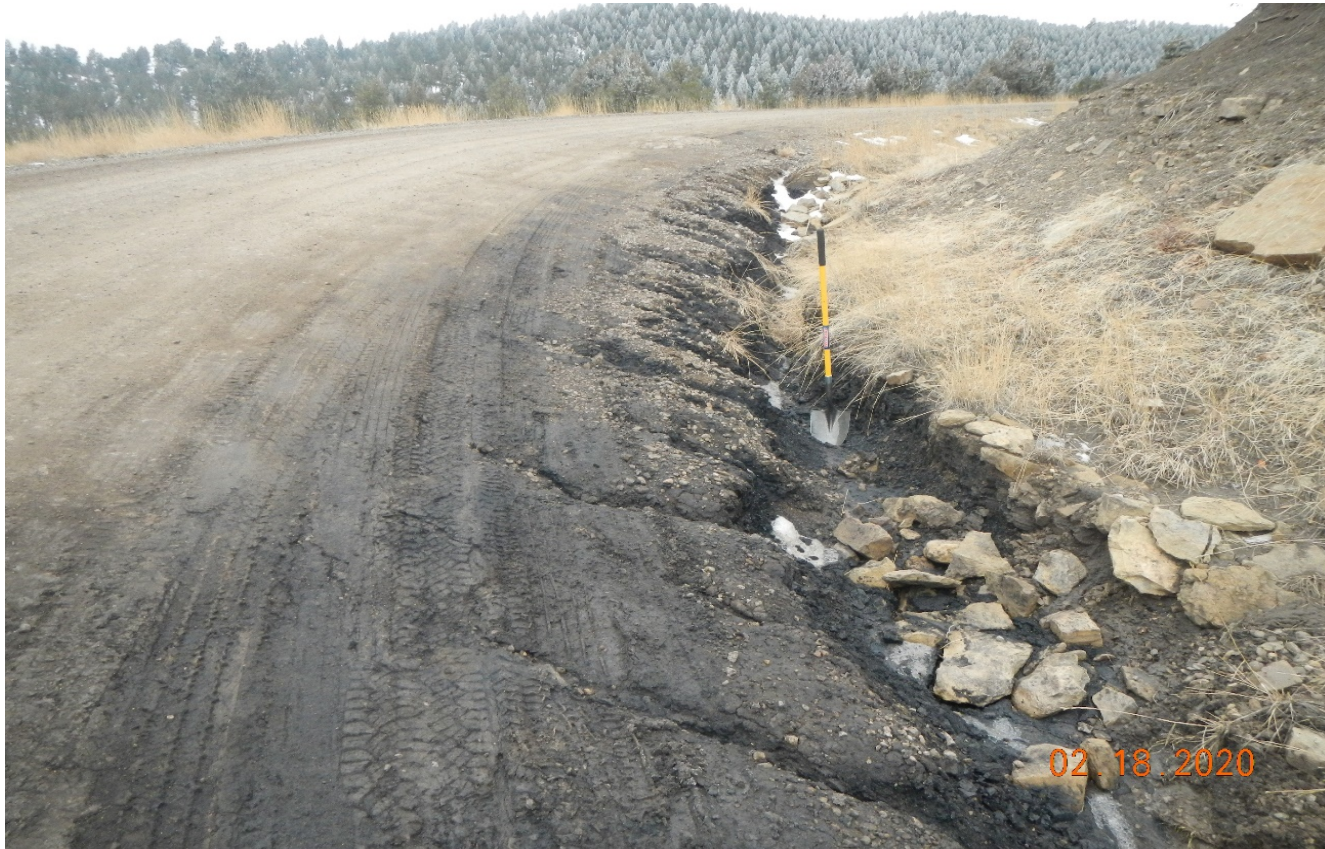
Photo 2. There is erosion occurring along the main road and no BMP's are installed to prevent erosion.
