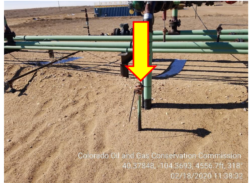
Photo 5 – Unmarked 1” Riser west of Compressor
