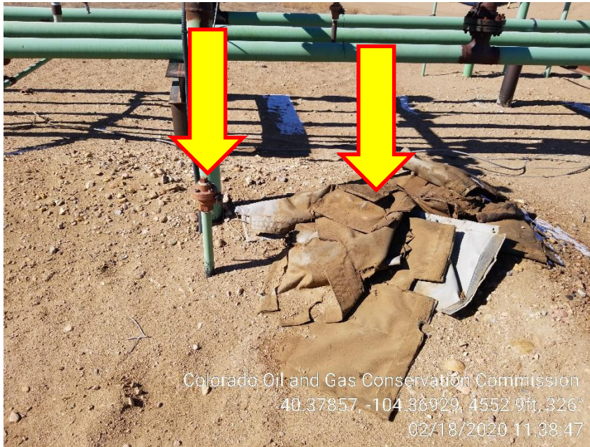
Photo 6 – Unmarked 1" Riser and trash west of Compressor
