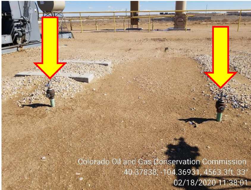
Photo 5 – 2” Unmarked Risers south of Compressor
