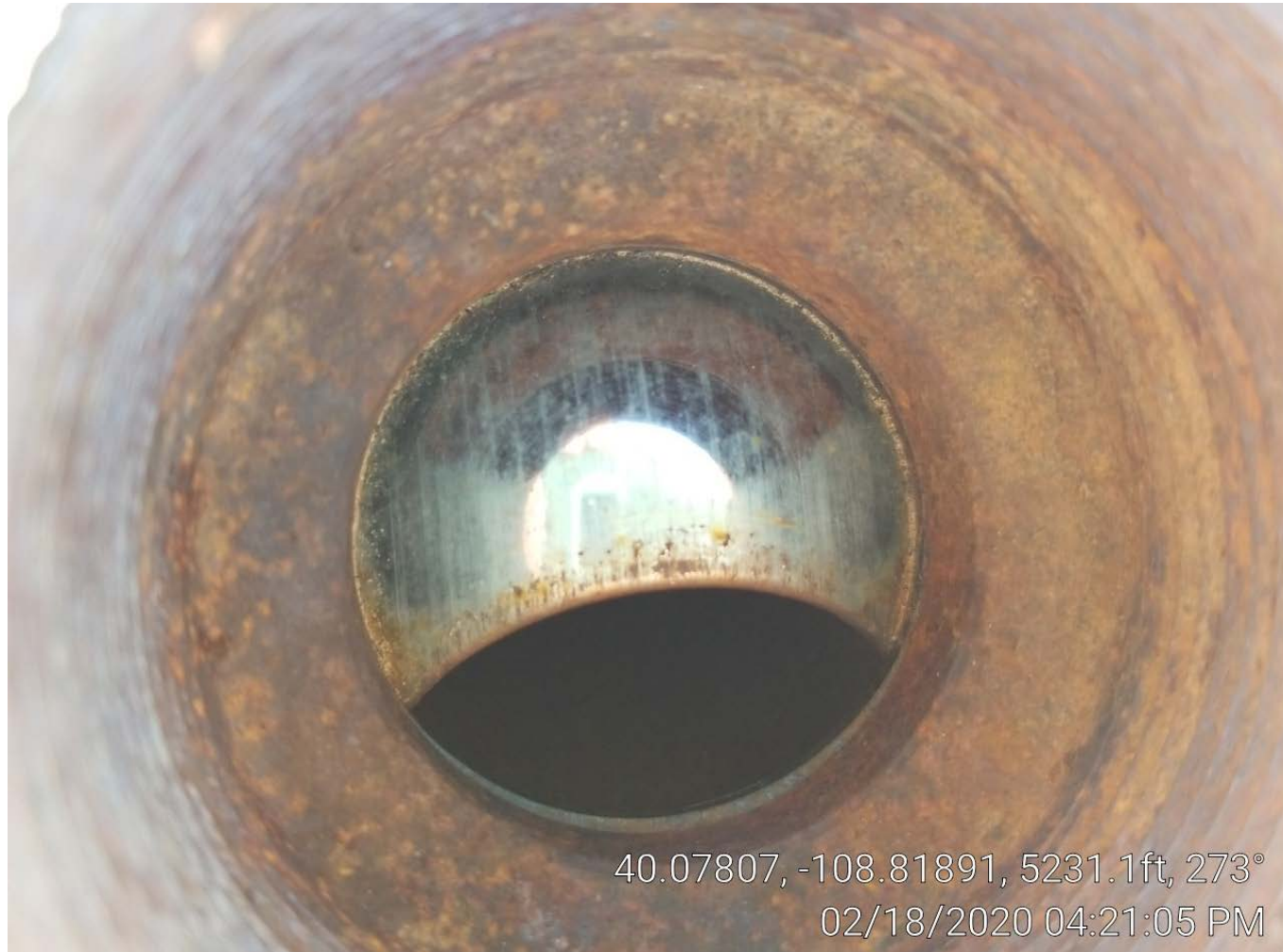
Photo 4. Casing valve.
