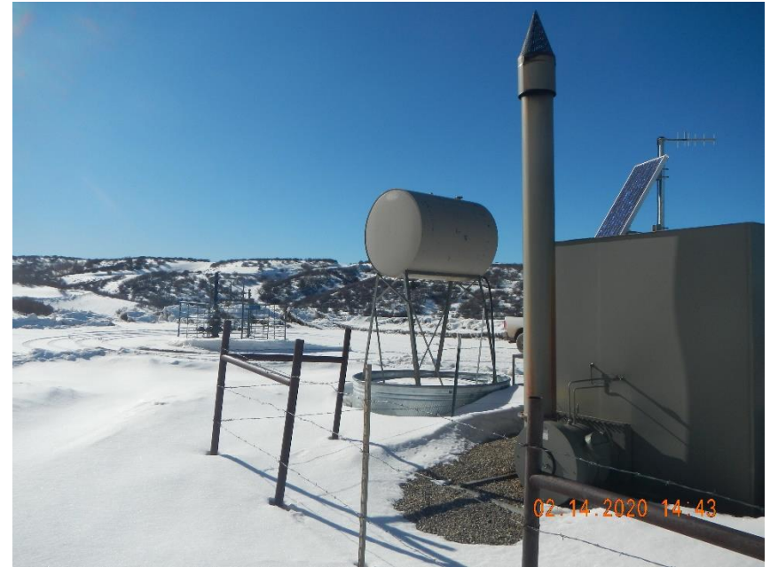
Capacity not on methanol tank at separator.
