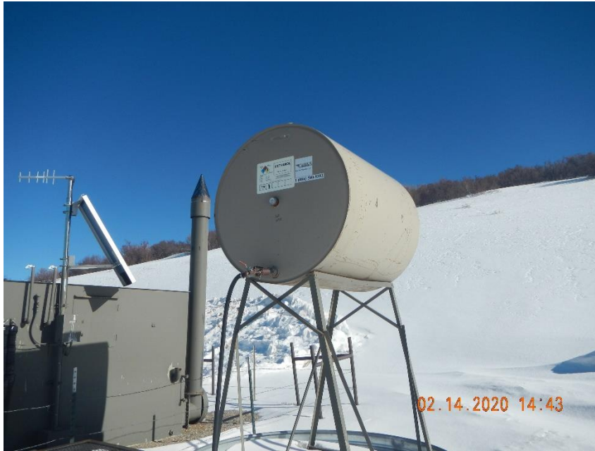
Capacity not on methanol tank at separator.
