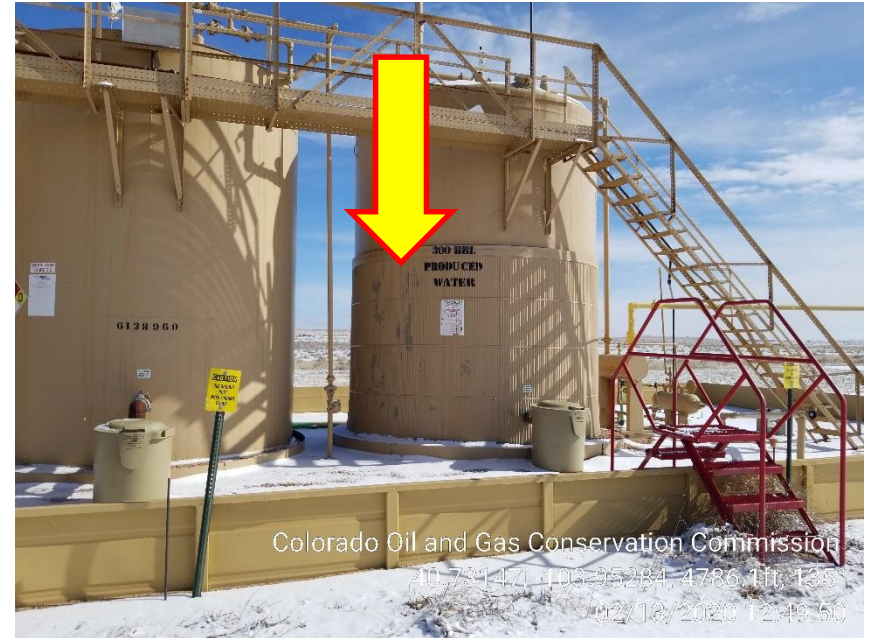
Photo 2 – Tank Missing NFPA Label
