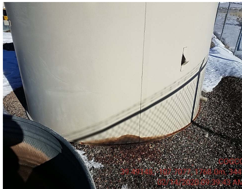
Tank is leaking
