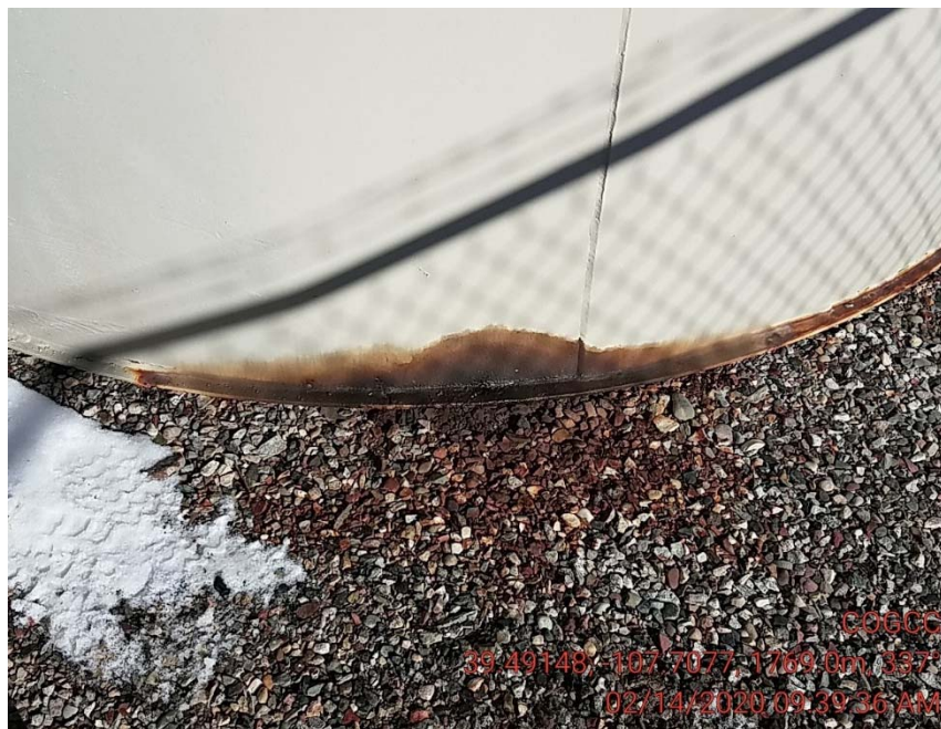
Tank is leaking
