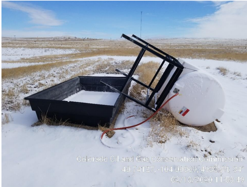
Photo 3 – Unused Chemical Tank and Containment. See photos. If still in use, please stand Chemical Tank backup and install wildlife netting on Secondary Containment.
