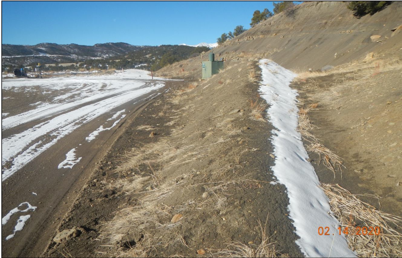
Photo 2. Facing toward the location. A berm is installed along the cut slope to contain erosion.
