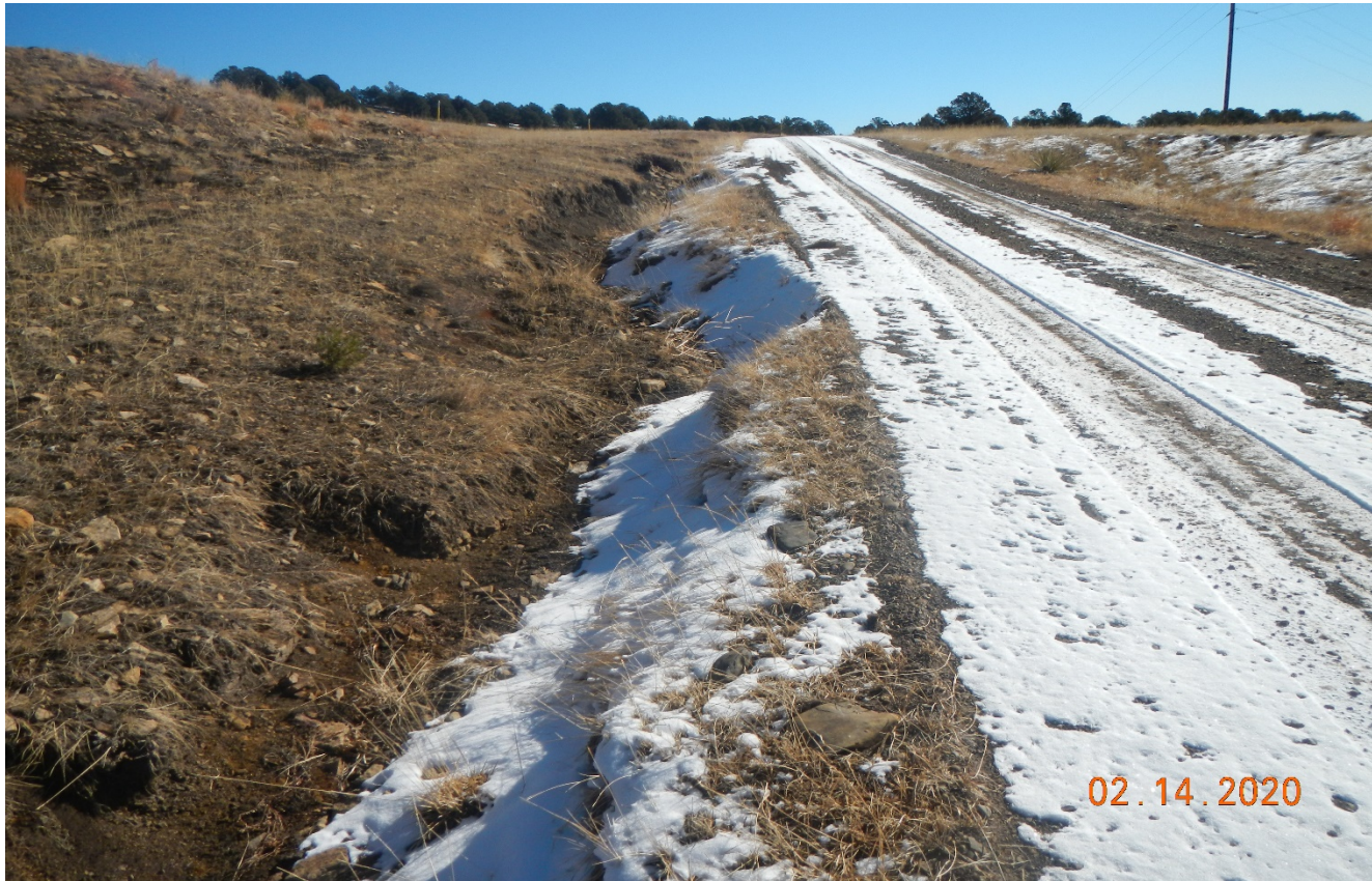
Photo 1. There is stormwater erosion which is occurring along the main road as it ascends the hill. BMP's need to be installed. Lat/Long:37.13882,-104.85030.
