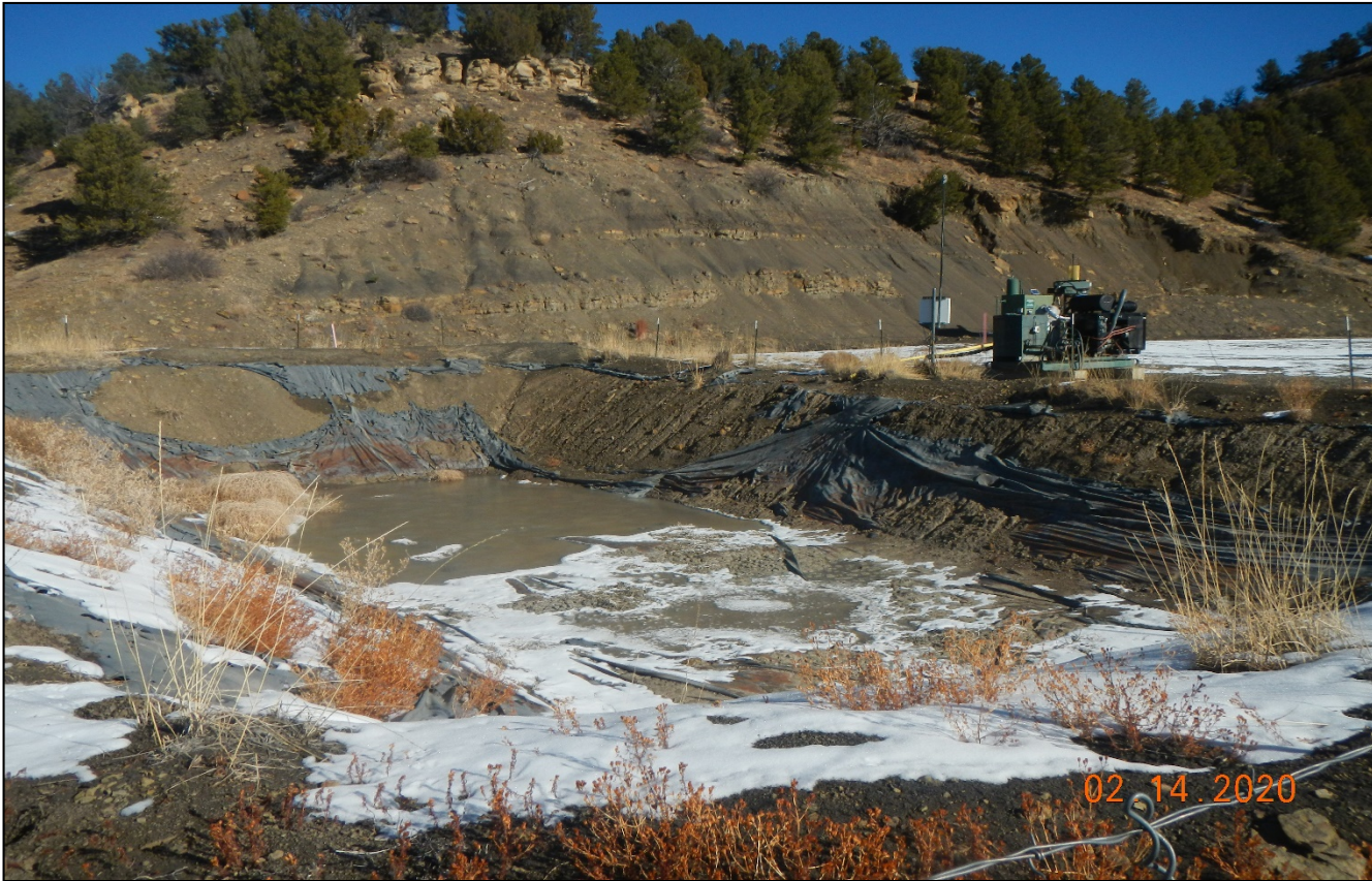
Photo 5. The pit liner is torn and degraded. There did not appear to be produced water in the pit at time of inspection.
