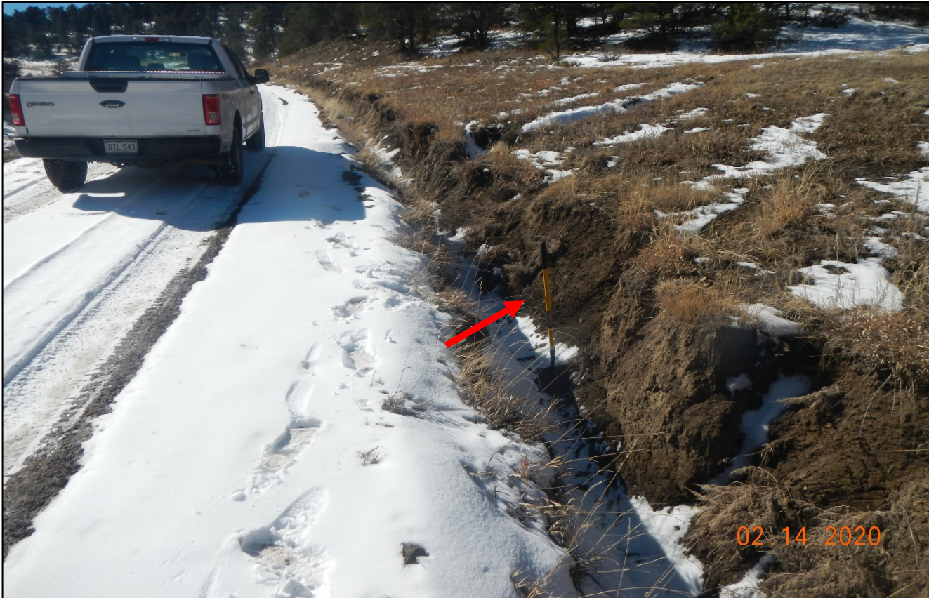
Photo 2. There is a deep erosion channel along the side of the main access to the location. Arrow points to 4.5 ft. shovel to show depth of erosion.
