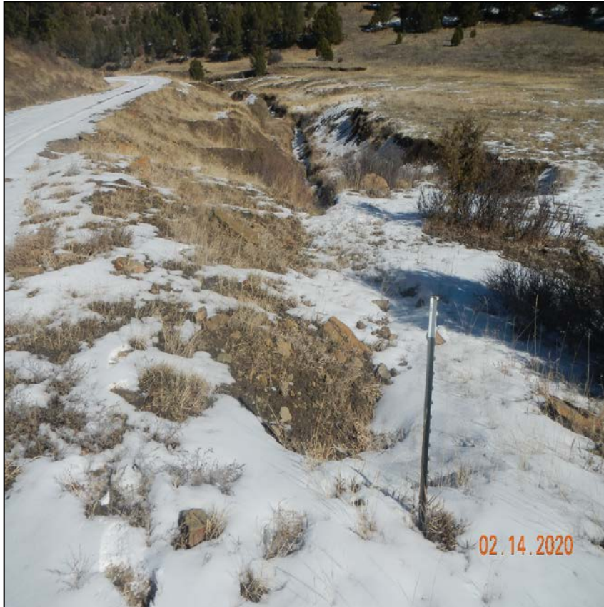
Photo 3. The stormwater outlet from this culvert is contributing to erosion of this gully. Lat/Long:37.14924,-104.86830.
