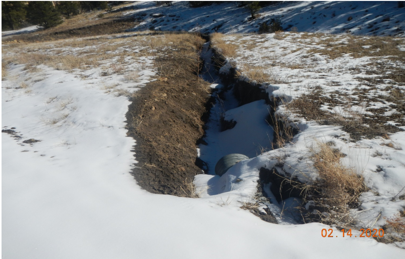
Photo 1. There a deep erosion channel at the outlet of the culvert along the main access road at Lat/Long:37.14466,-104.86788.
