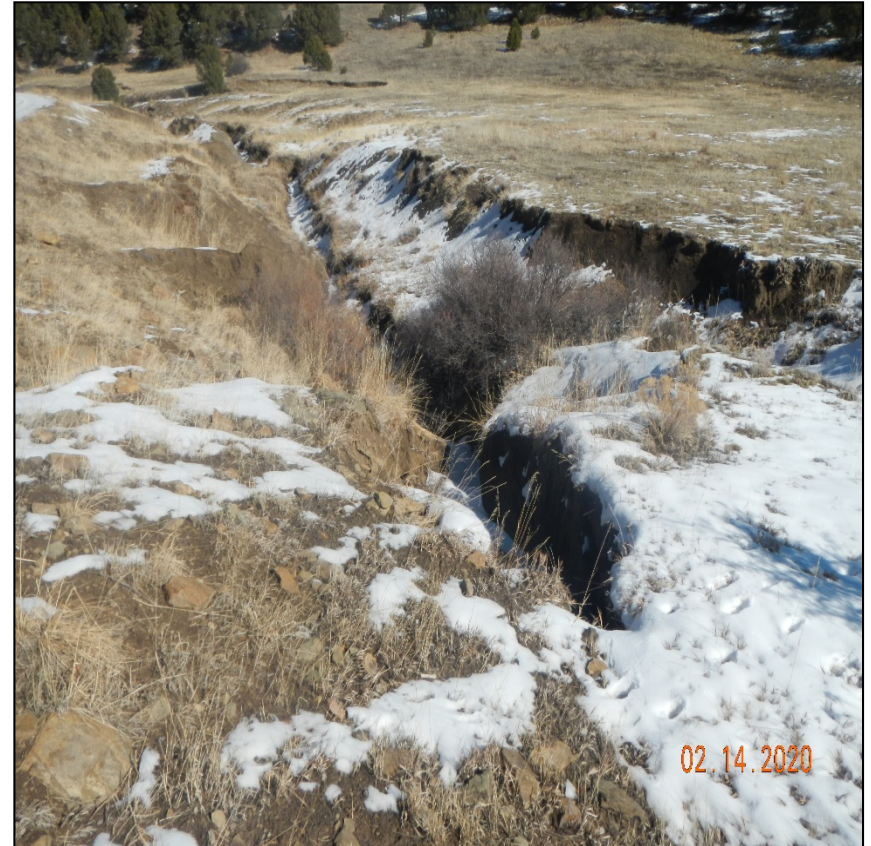
Photo 3. The stormwater outlet from this culvert is contributing to erosion of this gully. Lat/Long:37.14924,-104.86830.
