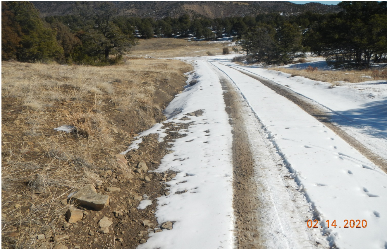
Photo 1. There is stormwater erosion which is occurring along the main road as it ascends the hill which is contributing to erosion further down the road. BMP's need to be installed. Lat/Long:37.14162,-104.86902.
