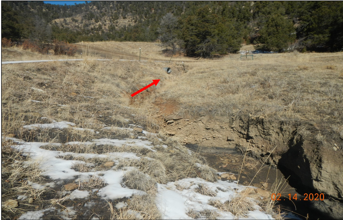
Photo 2. The culvert outlet which stormwater is direct from the Pacheco well sites is concentrating stormwater and causing erosion at this area Lat/Long:37.14117,-104.87398.
