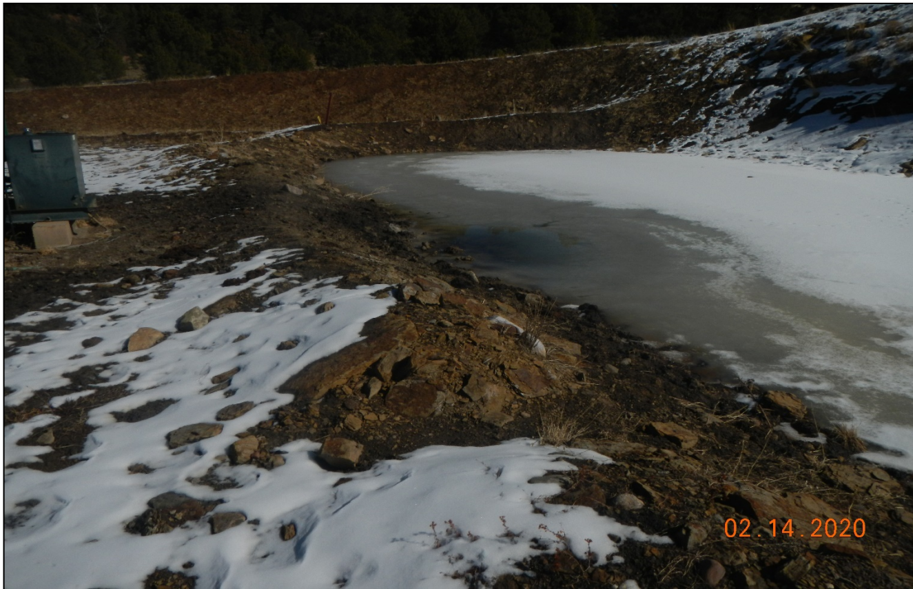
Photo 5. The water level at the pit is nearing 2 ft. freeboard.
