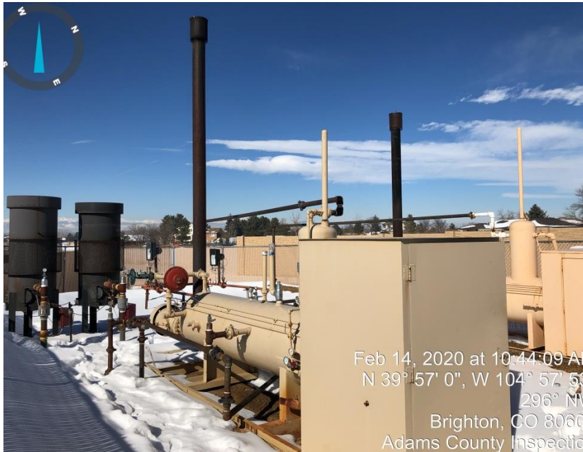
Photo#1 Separators/ECD's/Gas Meters
