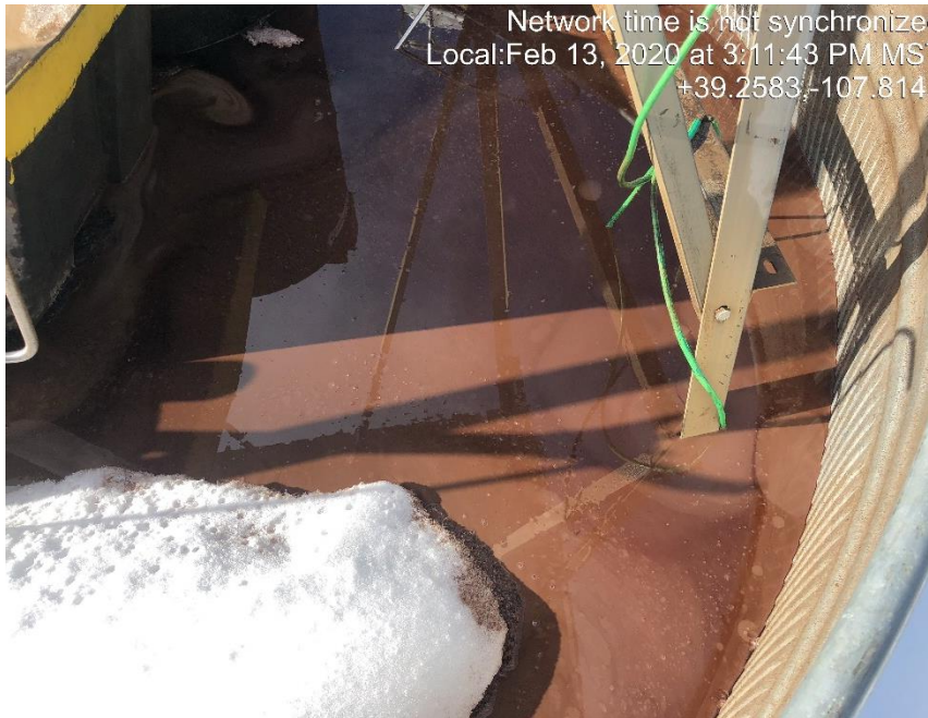
Photo #0594 Multiple containments with oily fluids inside them.
