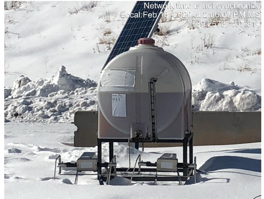
Photo #0585 Chemical tank by wellheads NFPA labels weathered and not legible.
