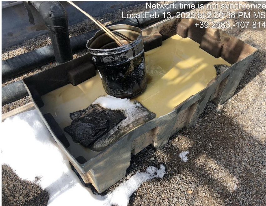
Photo #0587 Multiple containments with oily fluids inside them.
