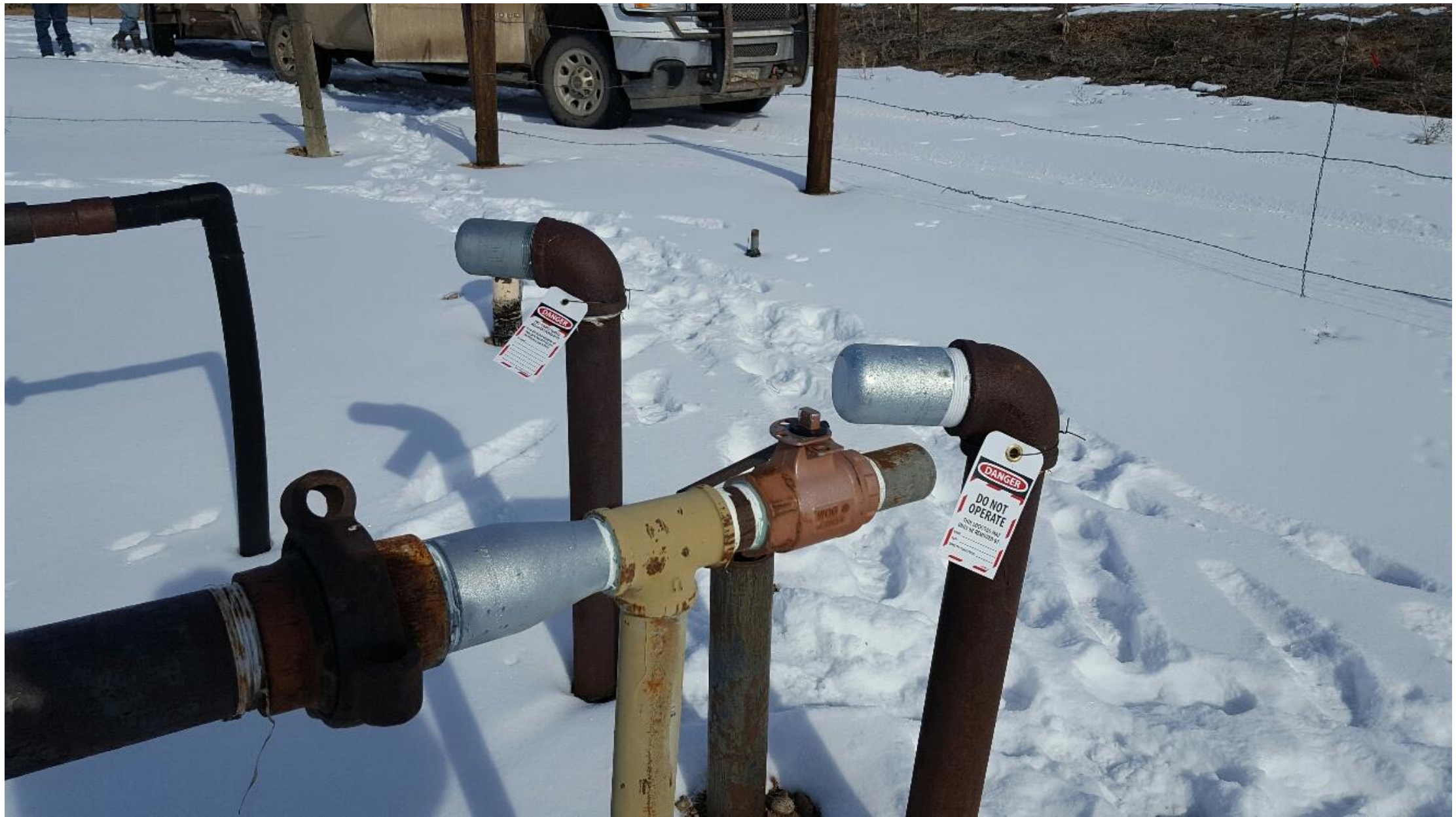
Figure #5 Risers have been marked.
