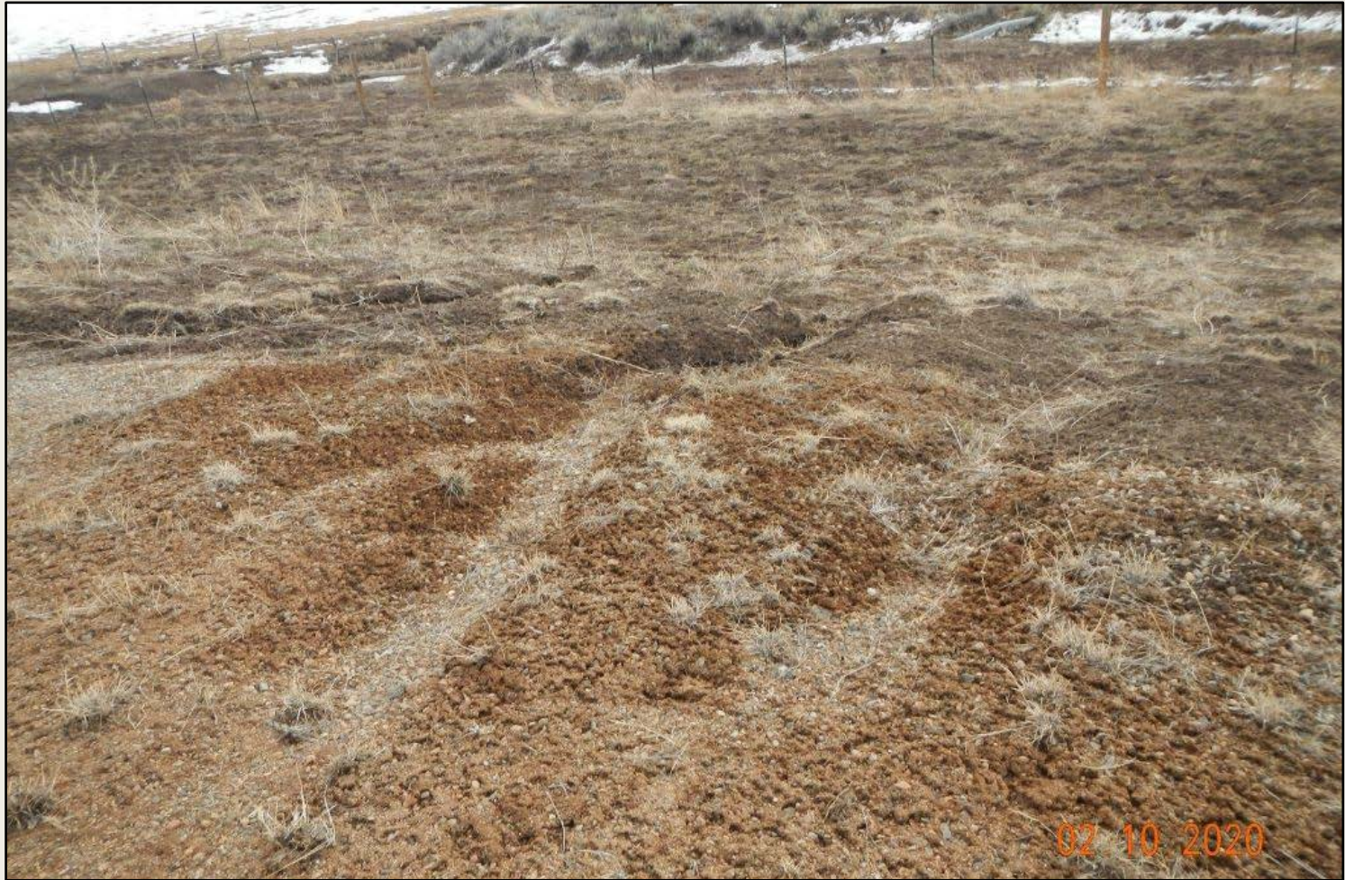
Photo 3. View of area within the southwestern fill slope where bare soils are not stabilized and rilling is evident.
