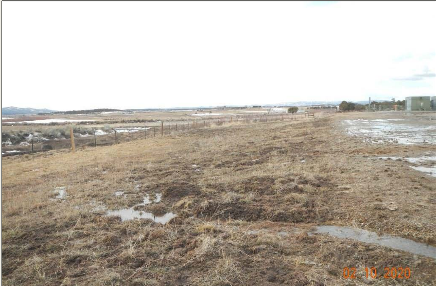
Photo 2. View of the southern project area from the southeastern corner facing westward. Vegetation is largely in a grazed/dormant condition at this time with perennial grasses largely not in identifiable condition. Stormwater erosion is occurring across the fill slope as grazed grasses are not sufficiently stabilizing the project area.
