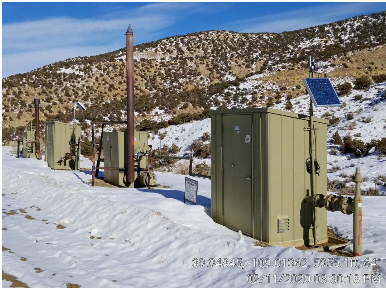
Photo 3. Separators & meter buildings.
