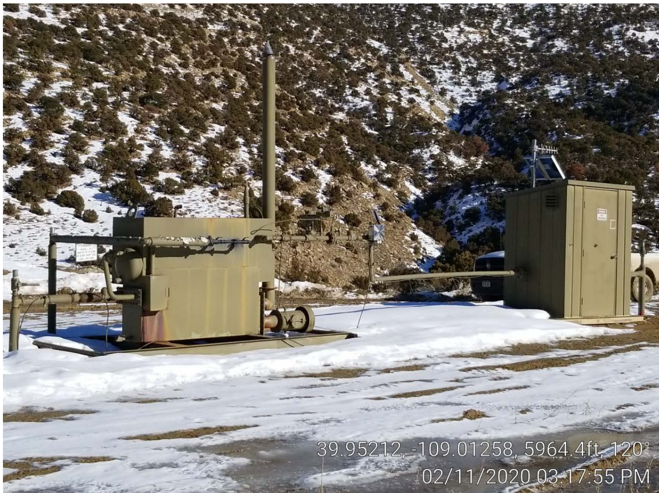
Photo 3. Separator & meter building.
