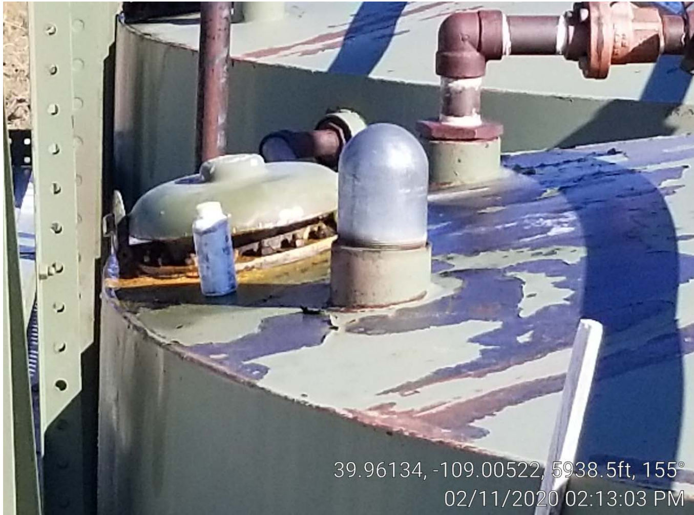
Photo 5. Gas venting out around edges of hatch on middle tank.
