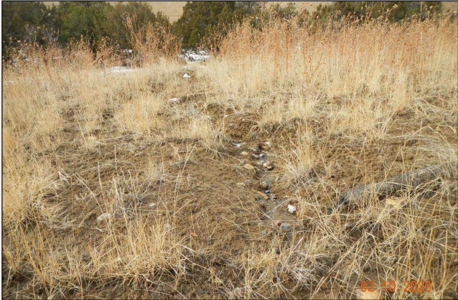
Photo 3. View of area within the western fill slope where snow melt is actively flowing off of the well pad, creating an erosional channel. Wattle is not functioning and is not an adequate BMP in this area.
