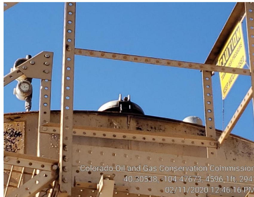
Photo #7 Broken thief hatch latch
