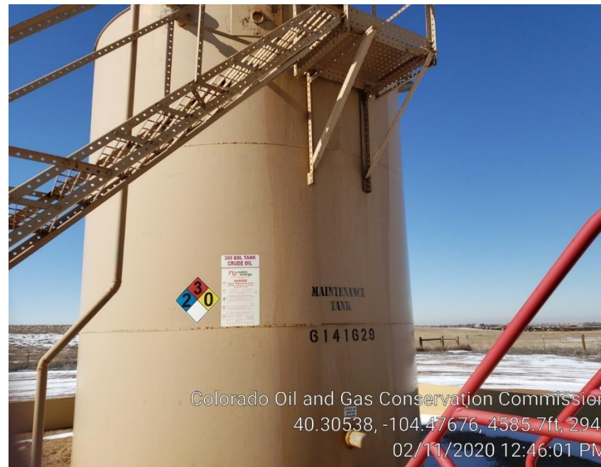
Photo #5 Maintenance tank oil stain down the side.
