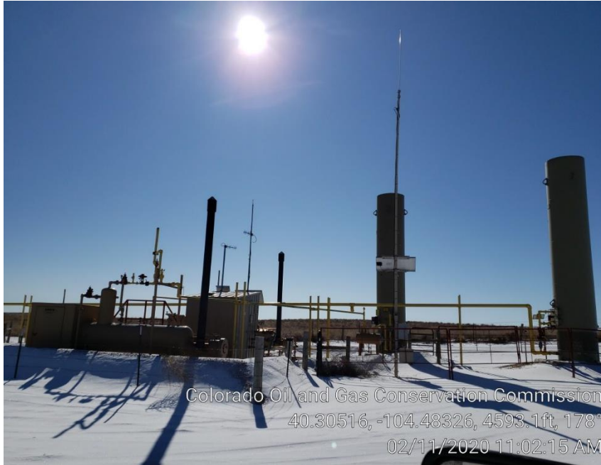
Photo #2 Separator, ECD's & Meter Runs
