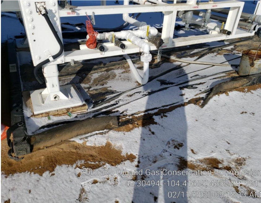
Photo #8 Tore Secondary Containment/ duck pond
