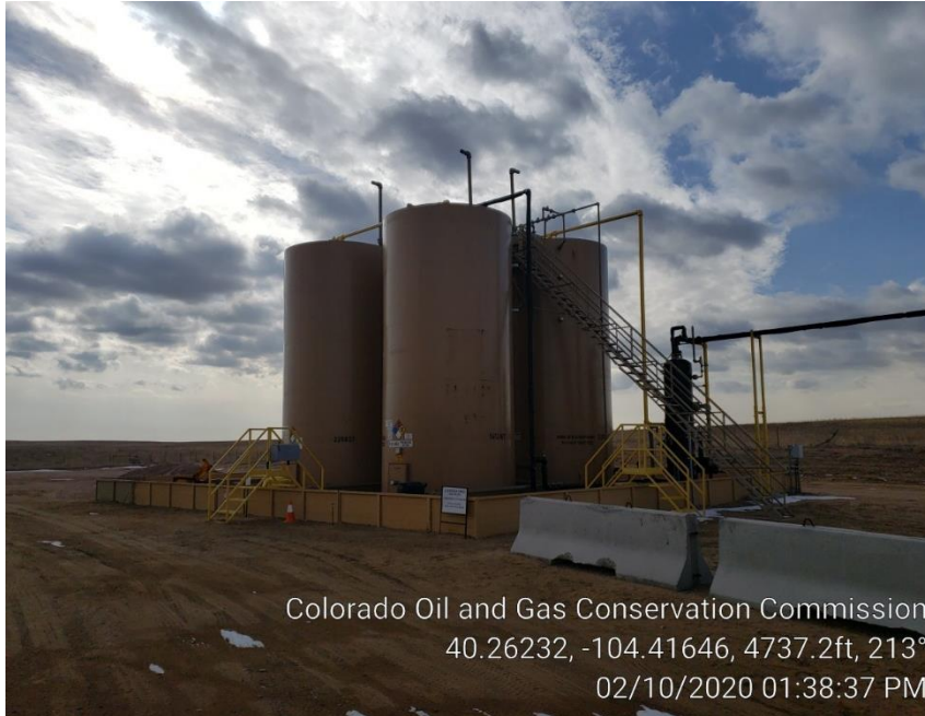
Photo #3 Tank Battery
