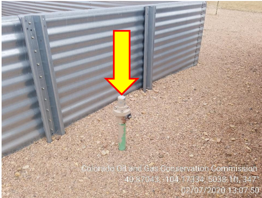
Photo 3 – Unmarked 2" Riser SE Corner of Tank Berm
