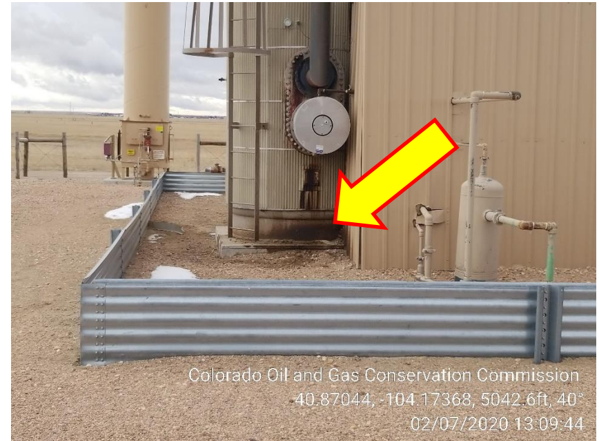
Photo 4 – Stained Soil at Heater Treater
