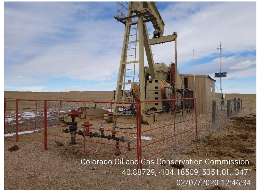
Photo 2 – Wellhead and Pumping Unit
