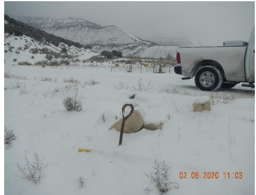
Anchor marker is down for anchor off edge of road.
