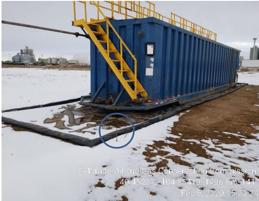
Photo 17: Tank appears to be grounded
