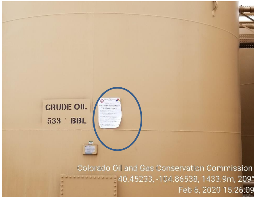
Photo 21: NFPA placard applied to tank
