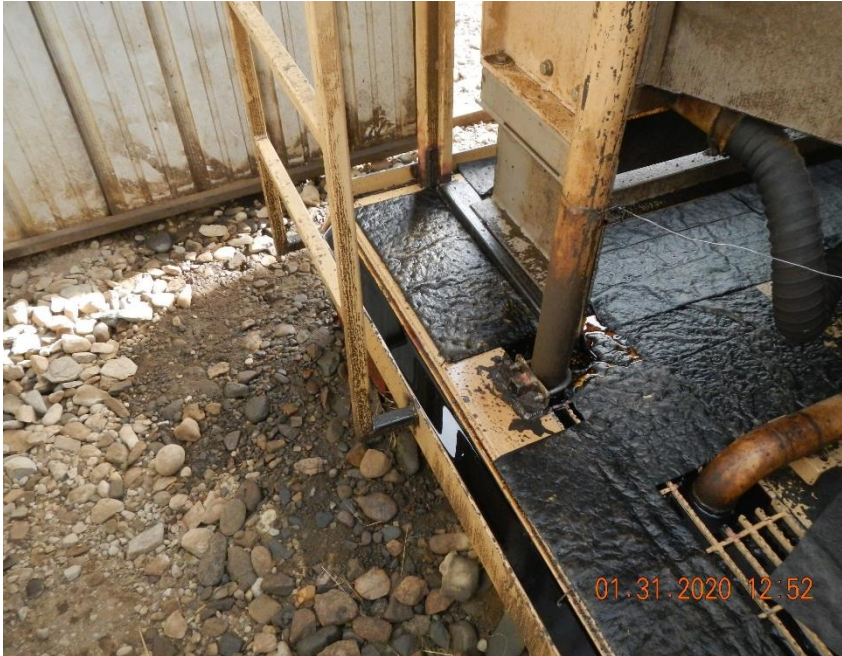
Saturated absorbent rags beneath equipment.
