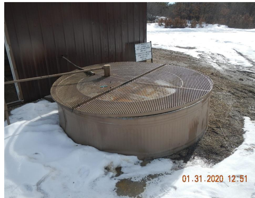
Unlabeled produced water vessel.
