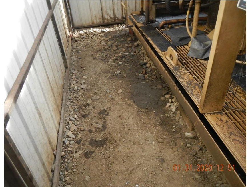
Stained soil along edge of compressor skid.
