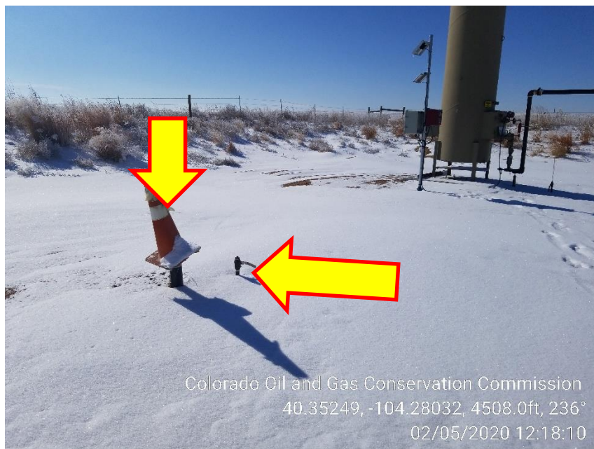
Photo 3 – Unmarked Risers
