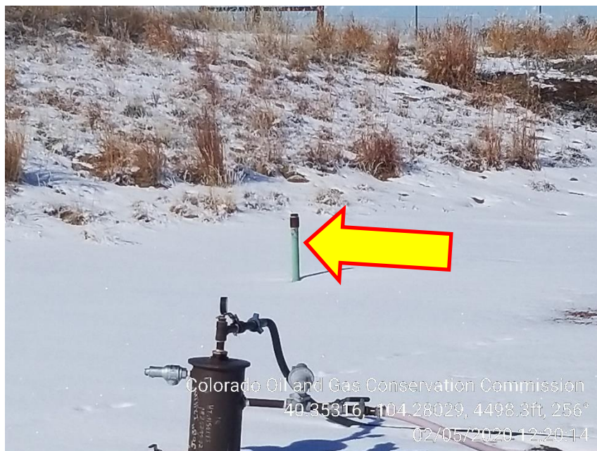
Photo 5 – Unmarked Risers
