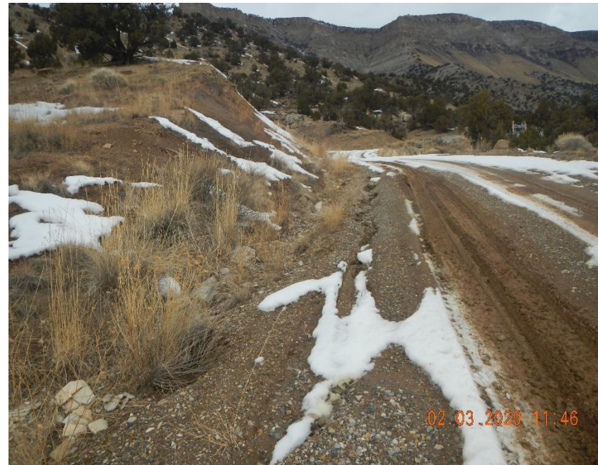
Road is rutting and ditches eroding into roadway.
